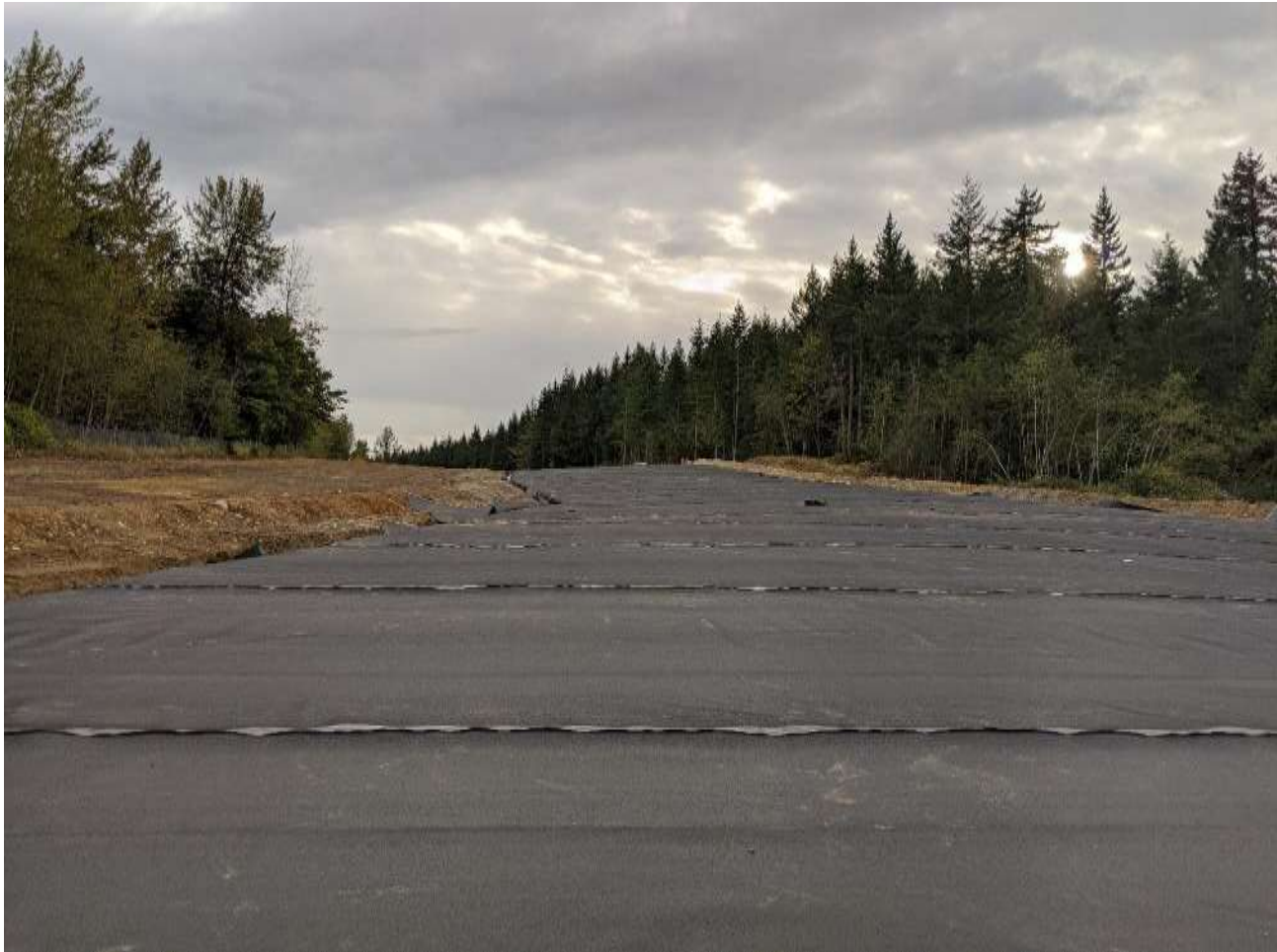
Photograph 4: Geomembrane liner deployed over Area 8.
