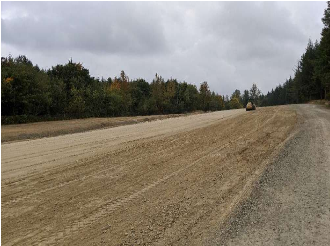
Photograph 2: Areas 7 and 8 regraded and being rolled in preparation for liner installation.
