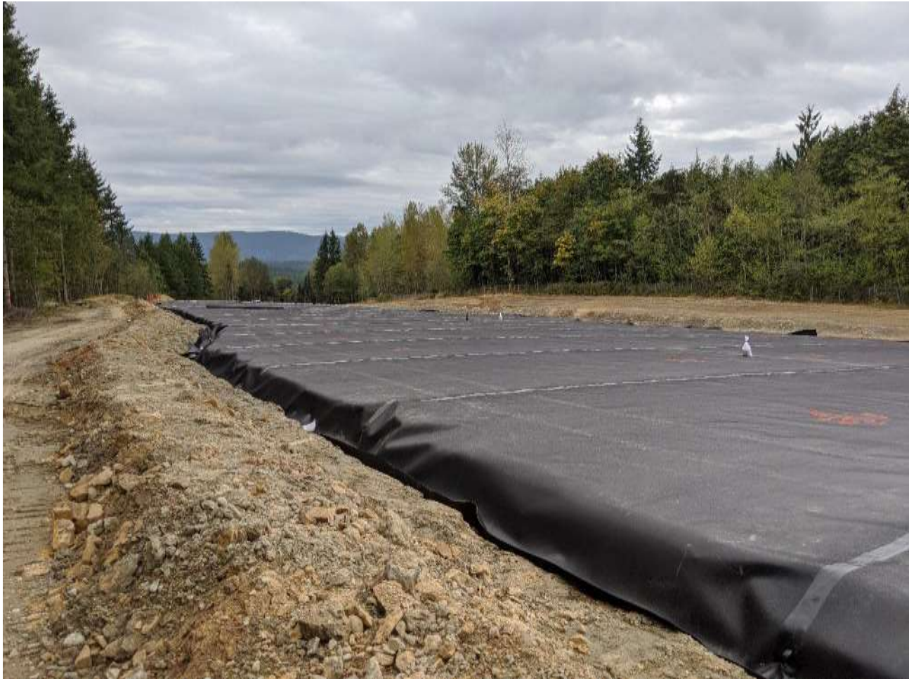
Photograph 3: Geomembrane liner deployed over Area 7.
