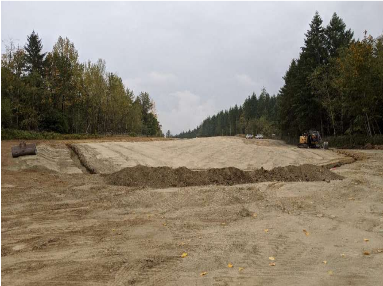
Photograph 1: Anchor trenches dug and Area 8 subgrade rolled in preparation for liner installation.
