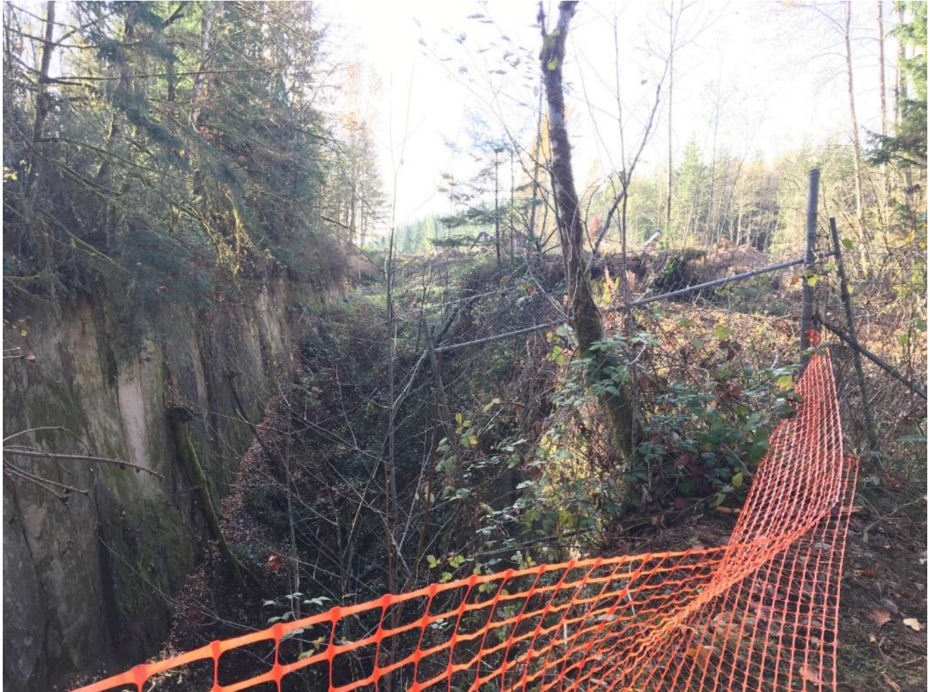
Photo 1 – Area 9, November 15, 2018 (looking south from northern tip)
