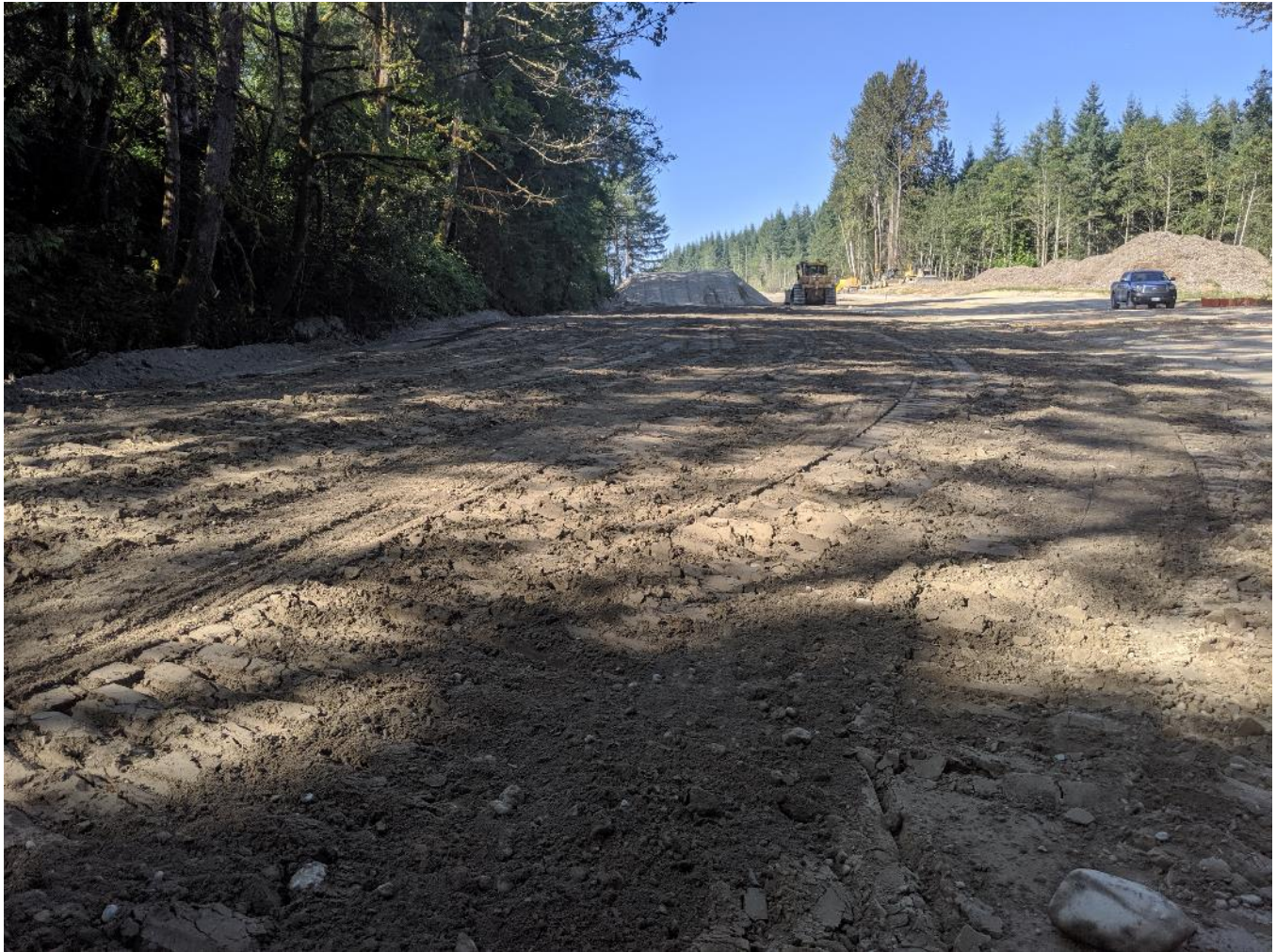
Photo 2 – Area 9, August 5, 2019 (looking south from northern tip)
