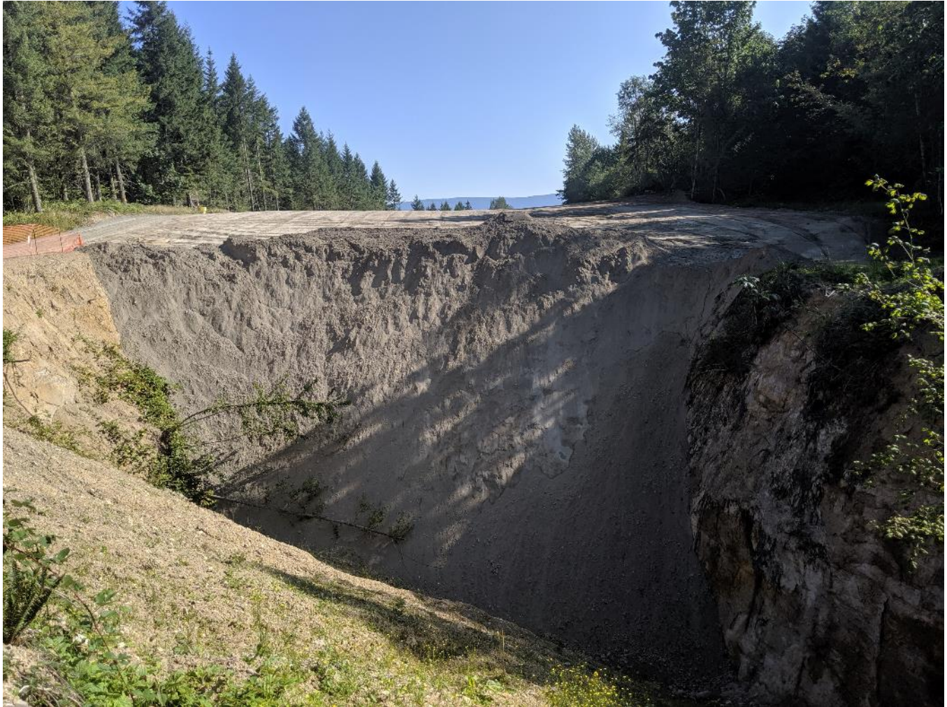
Photo 8 – Area 6 buttress, August 5, 2019 (looking north from southern tip)
