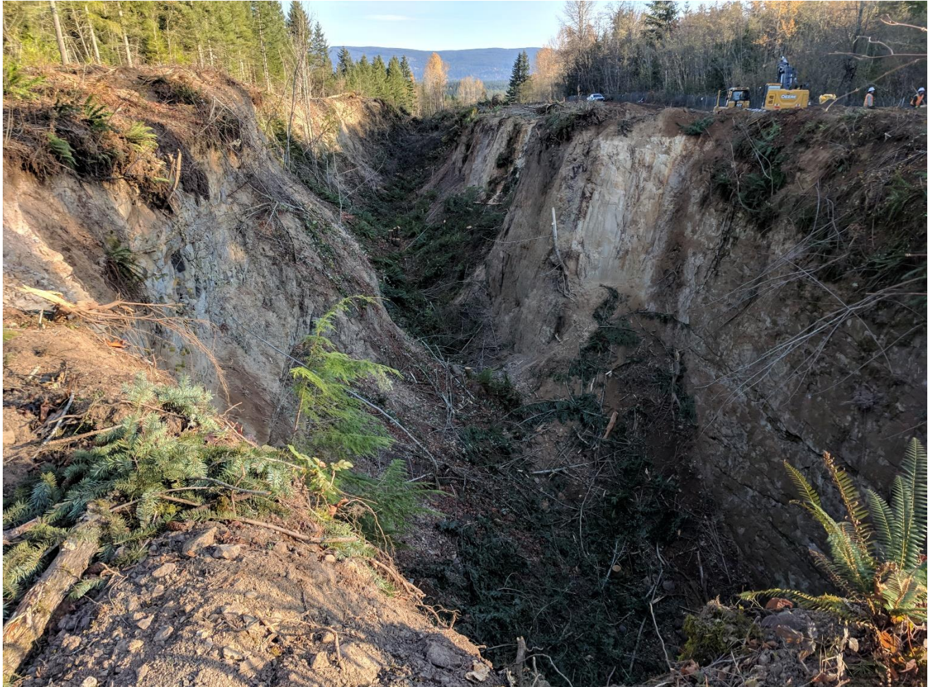
Photo 7 – Area 7, November 20, 2018 (looking northeast from southern tip)
