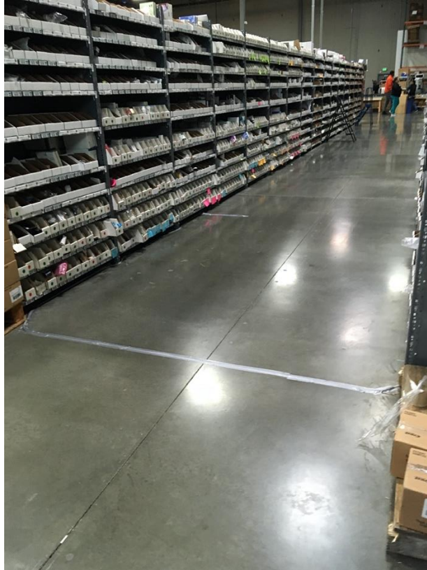
Photograph 1. Tubing installed at VP-7 to measure cross-slab differential pressure.
