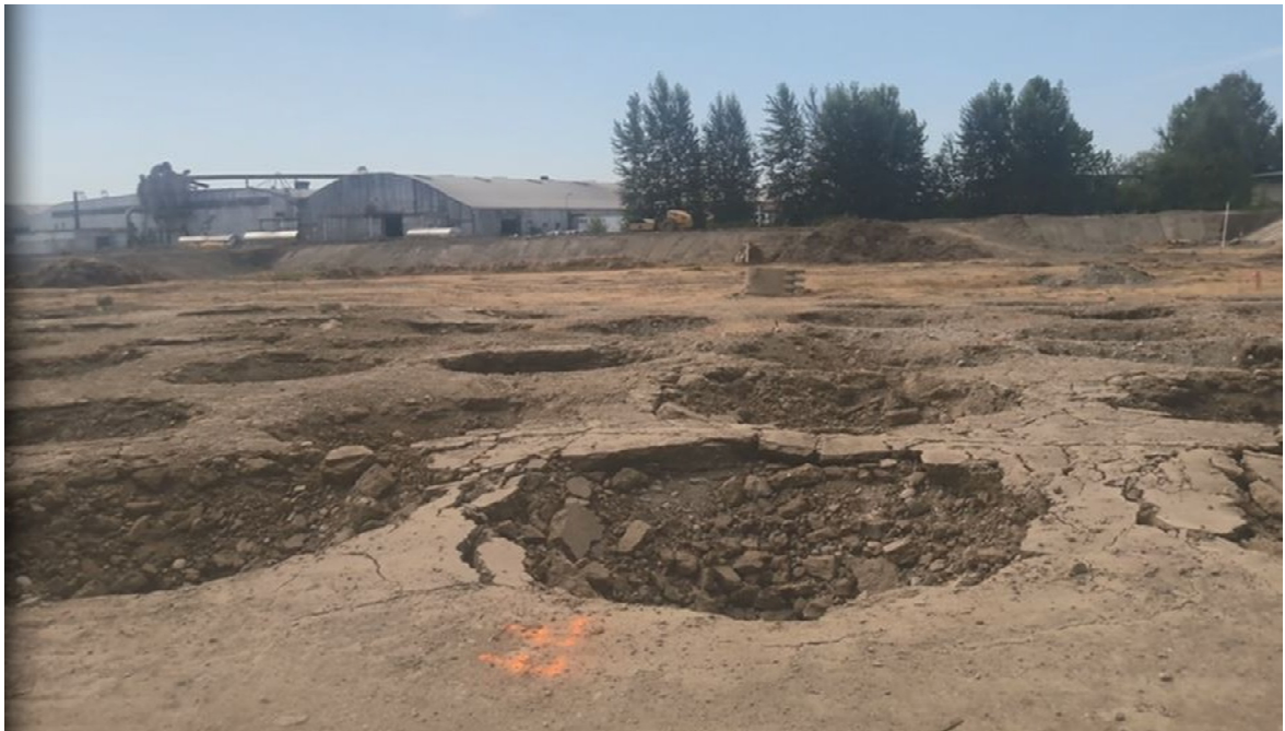
Photograph 2. Dynamic Compaction Impact Craters. Looking South
