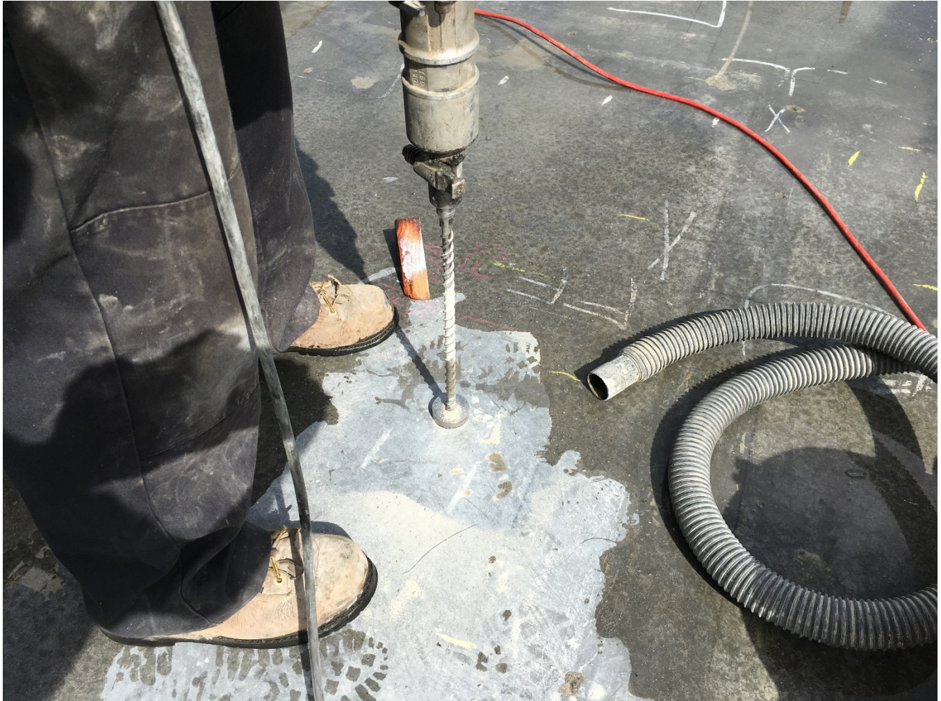
Installation of a Vapor Pin.
