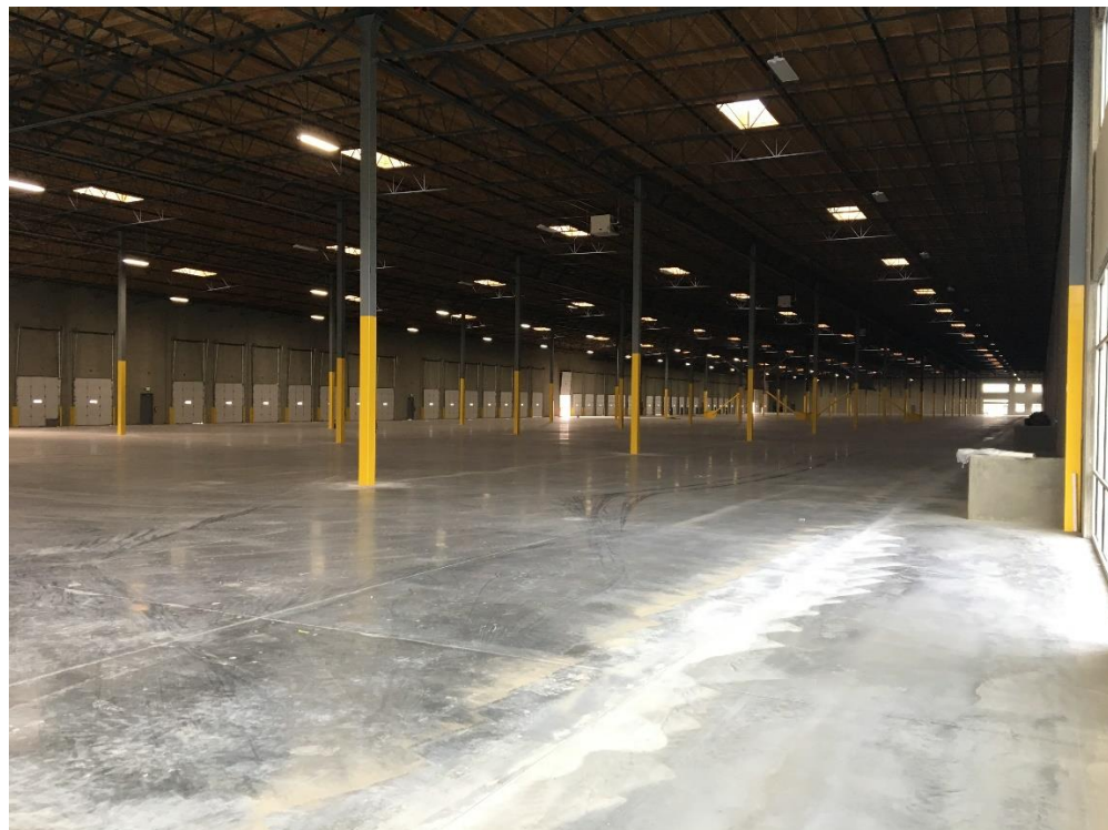
Photograph 6. Building A interior; northeast corner facing west.
