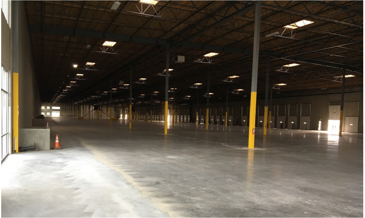
Photograph 11. Looking East in finished floor slab of Building A.
