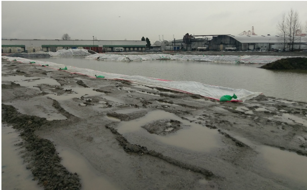
Photograph 5. Wet site conditions during initial methane and VOC vapor survey in April 2018. Stormwater Pond in Background, Looking North
