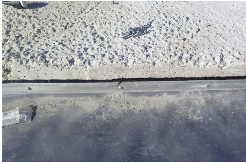
TYPICAL BATTEN STRIP SEAL PHOTO SCALE: NTS
