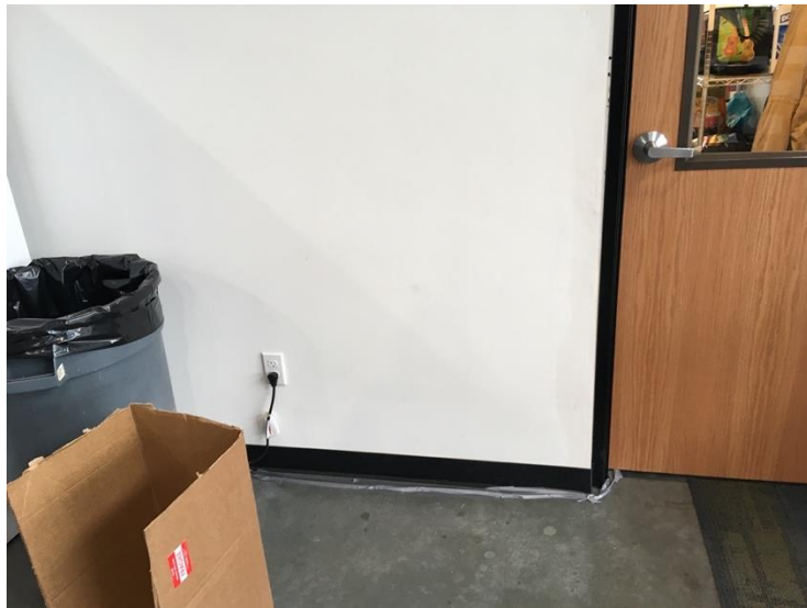
Photograph 3. Tubing run to Building A break room enclosure to measure differential pressure.
