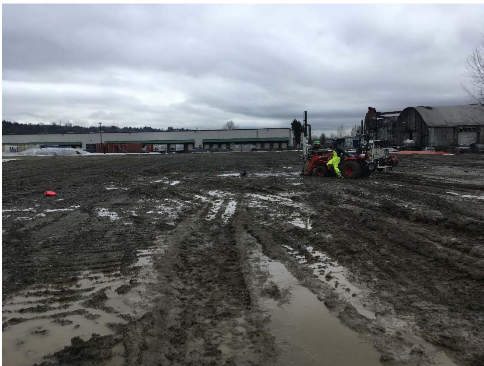
Caption: Drilling on building B pad, muddy conditions
