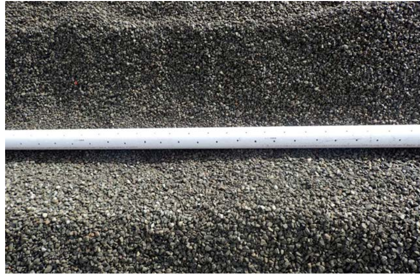
TYPICAL PERFORATED COLLECTION PIPE PHOTO SCALE: NTS
