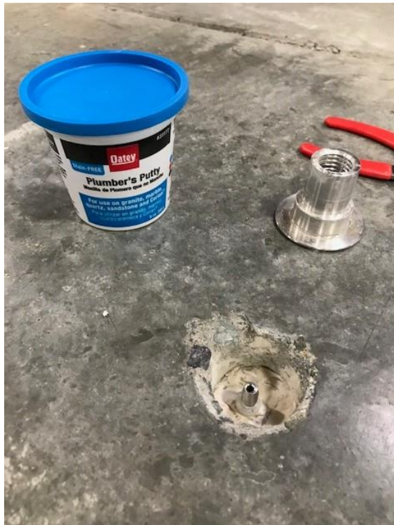
Photograph 7. Placement of additional seal to re-sample VP-3 after failed leak test.
