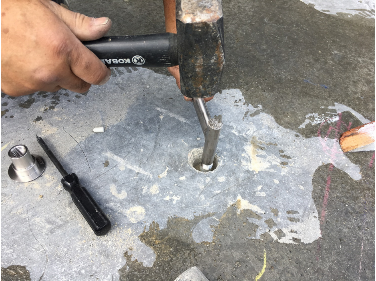
Hammering in Vapor Pin VP-14.
