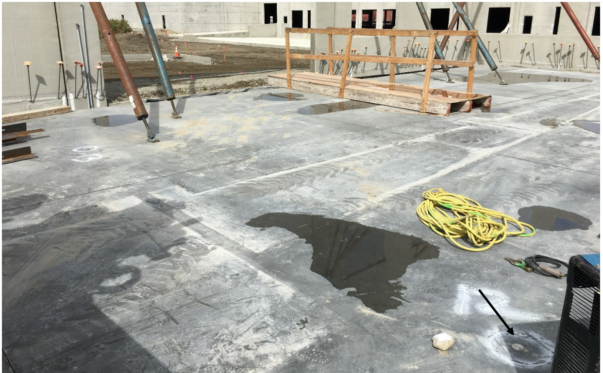
Photograph 14. Vapor Points VP-12 and VP-13 after installation.
