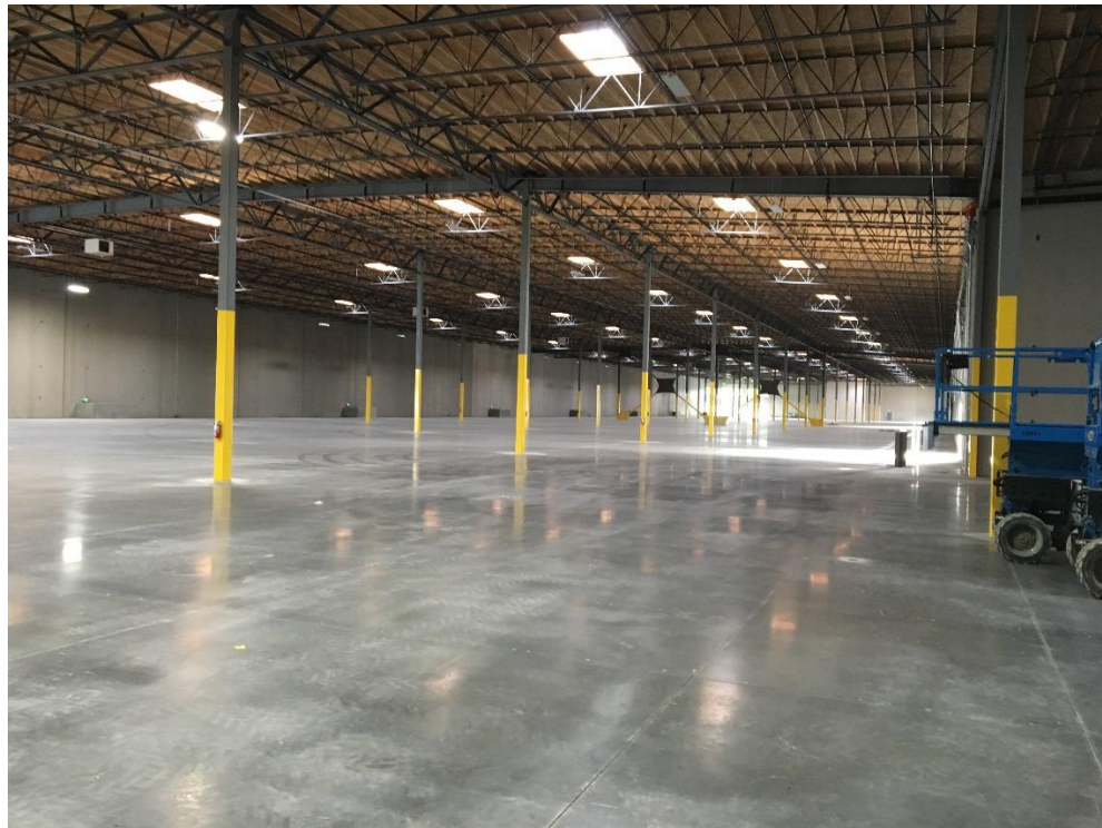
Photograph 10. Building A interior; southwest corner facing east.
