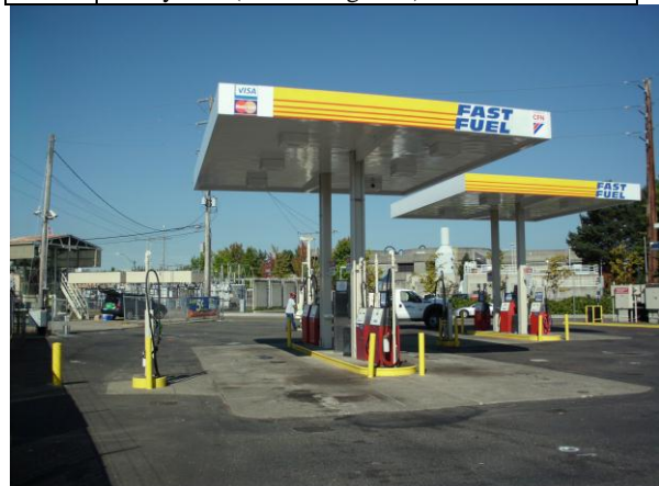
Photo #10: View of the Fast Fuel Cardlock facility, operated by Acme Fuel (looking to the north).
