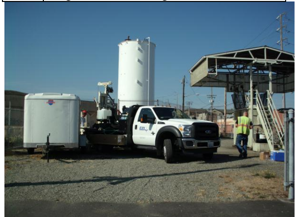
Photo #6: View of direct push probe drilling at boring B-3 (adjacent east of bulk fuel tank/spill area). View looking west.
