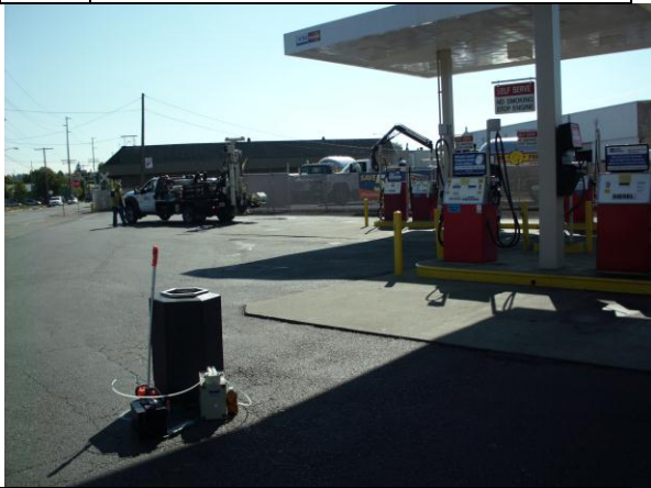
Photo #17: View of drilling at B-11, adjacent south of western dispenser island. Note groundwater sampling setup at B-9 in foreground.
