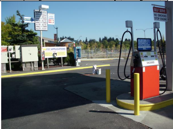
Photo #15: View of peristaltic pump (in background) set up to collect grab groundwater sample at boring B-9, adjacent east of eastern dispenser island.
