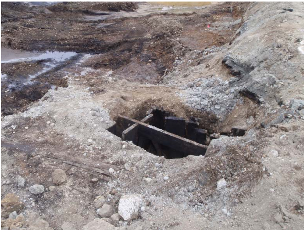
Photo 6 – Old wooden catch basin exposed on September 13, 2010 (looking west).
