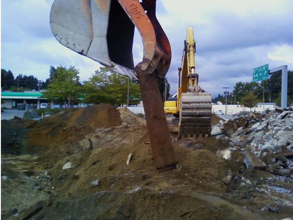
Photo 5 – Removing the hydraulic lift on September 7, 2010 (looking north).
