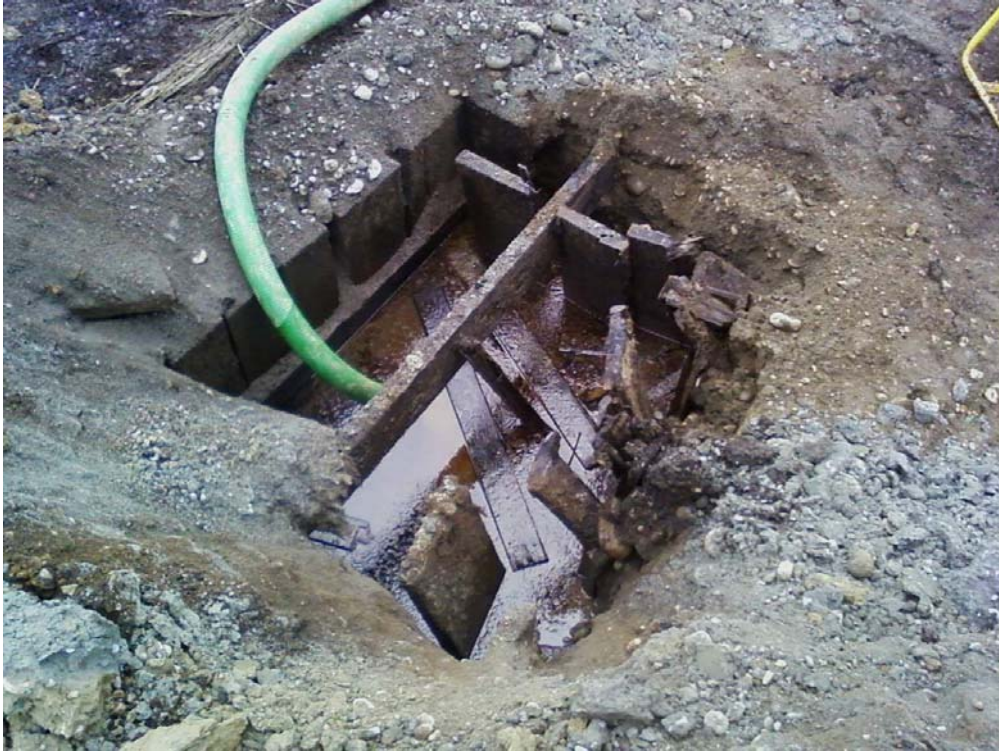
Photo 7 – Pumping water and oil out of old wooden catch basin on September 14, 2010.
