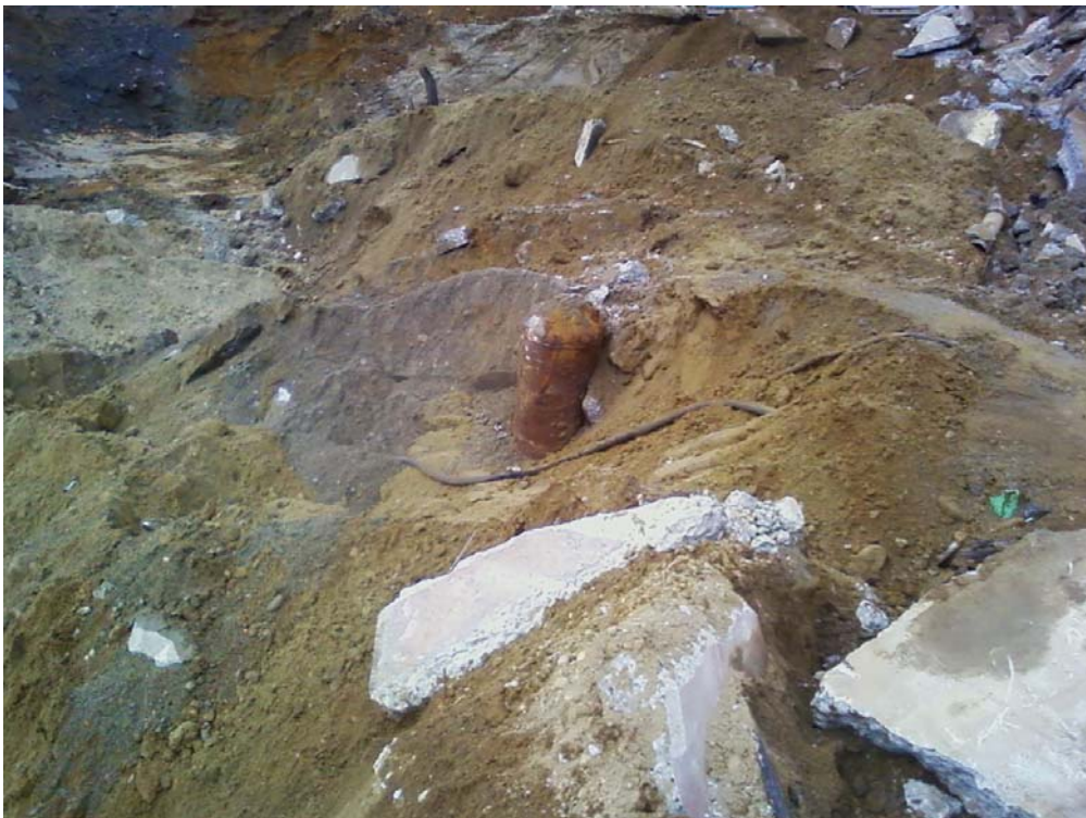
Photo 4 – Old hydraulic lift exposed on September 7, 2010.
