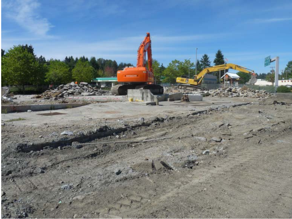
Photo 1 – Removing building foundations on September 2, 2010 (looking to west).
