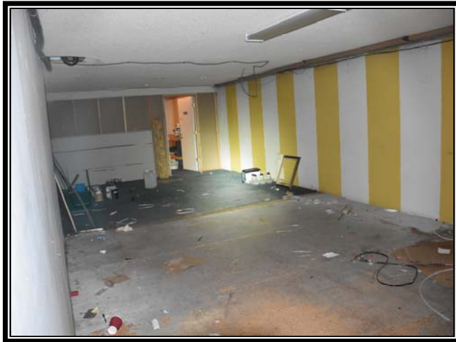
Photograph #13: 4/04/2019 Interior view of clubhouse basement.
