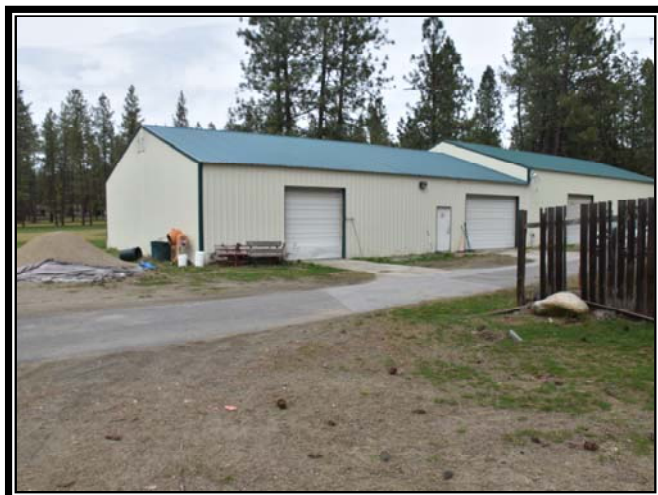
Photograph #18: 4/04/2019 View of maintenance garage looking north.
