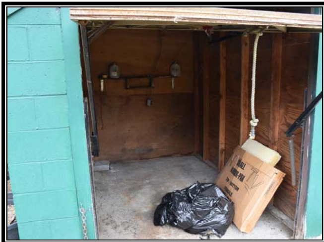
Photograph #17: 4/04/2019 Typical interior view of cart barn garage stall.
