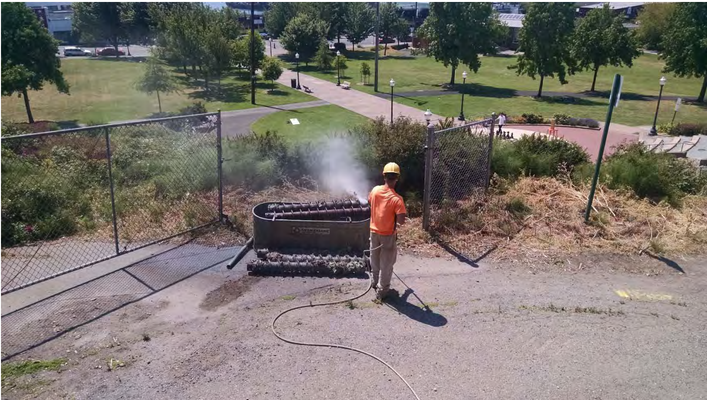
Pressure-washing the auger bits between borings.
