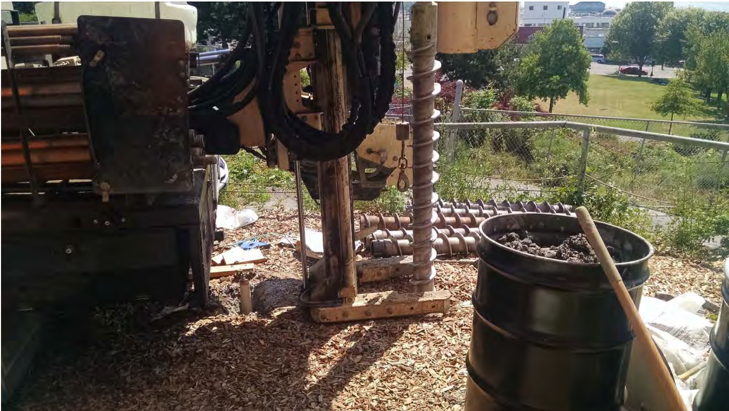
View of hollow-stem auger drilling in preparation of MW-1.
