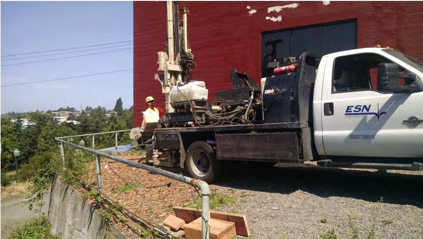
View of boring location SB1 (MW-1), looking northwest.
