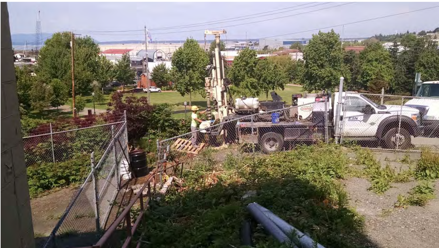
View of boring location SB3, looking west.
