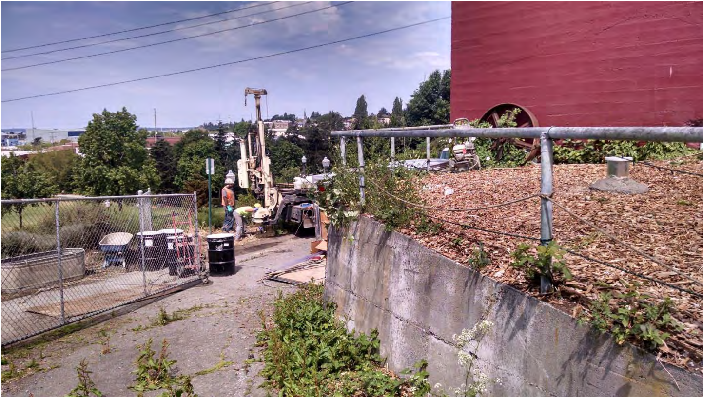
View of boring location SB4, looking northwest.
