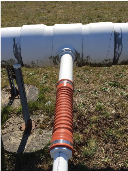
N-12 after 12"x3" Tee Replacement
