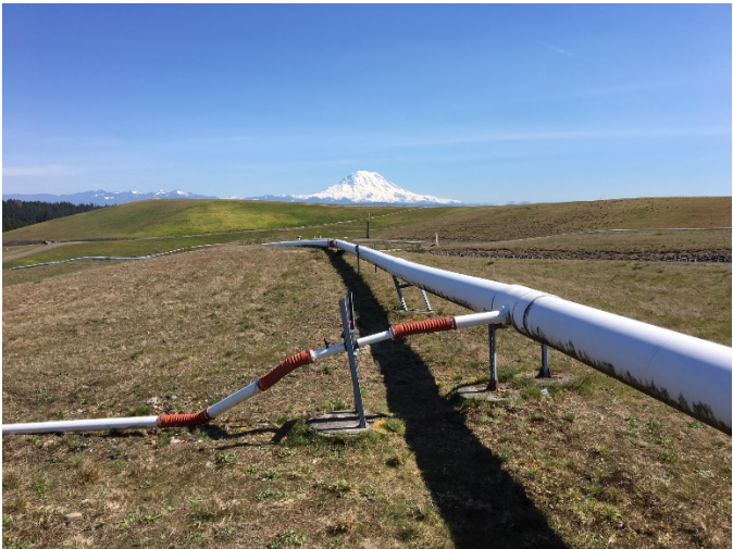
N-12 after 12"x3" Tee Replacement
