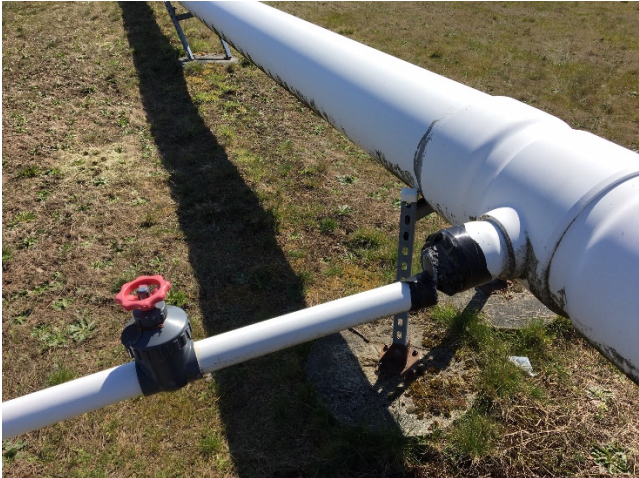
N-12 prior to 12"x3" Tee Replacement
