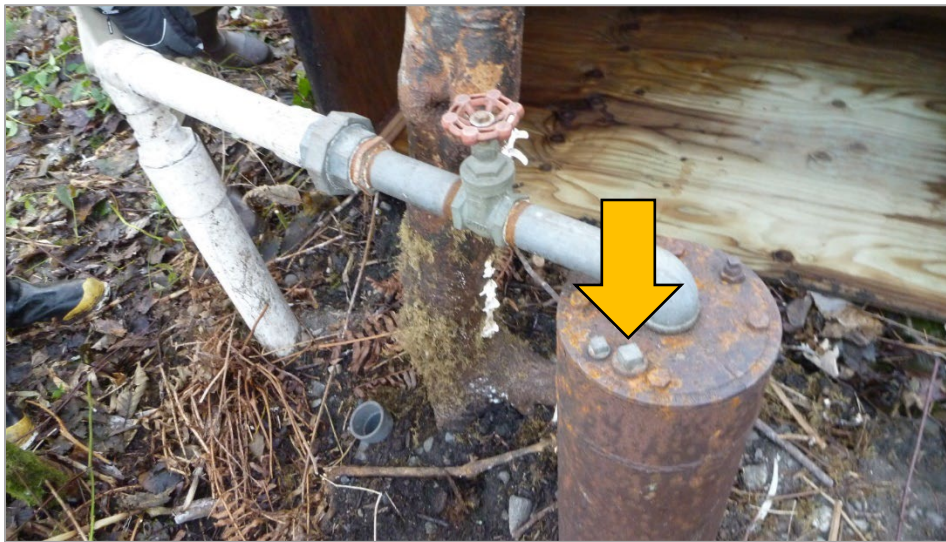
Figure 5: Arrow shows measuring point on a water supply well with access port (©2013, WA Dept. of Ecology).
