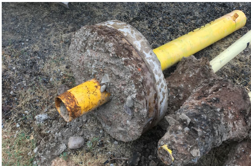
Figure 6: Well outer protective casing and monument removed for replacement with flush-mount monument. Requires a new measuring point (©2018, WA Dept. of Ecology).
