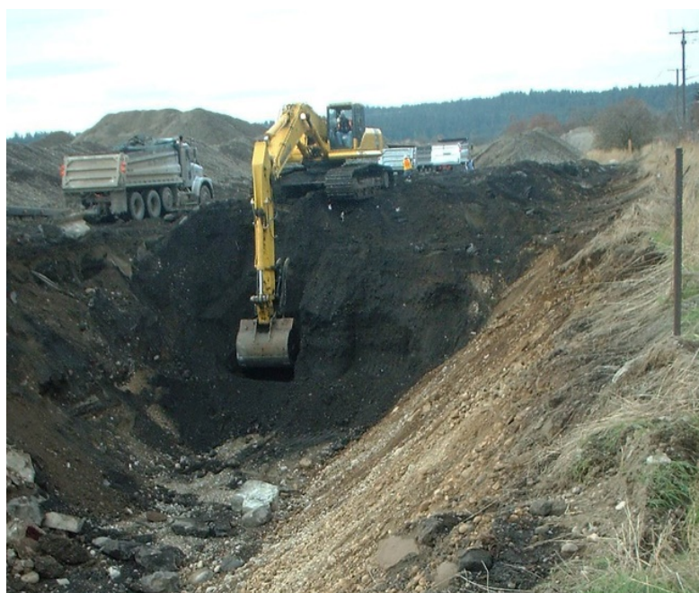
Figure 2. Removing contaminated material from an ash trench at Kendall Yards.
