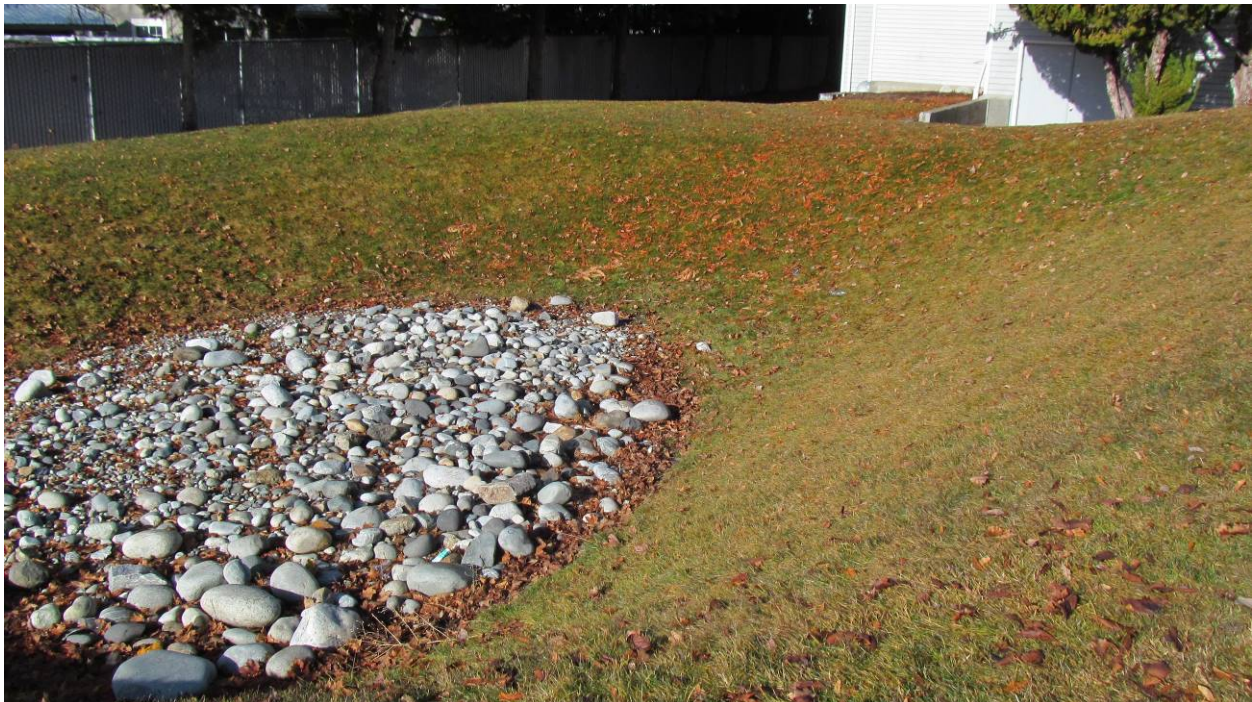
Photo 4: Stormwater Swale - from east
