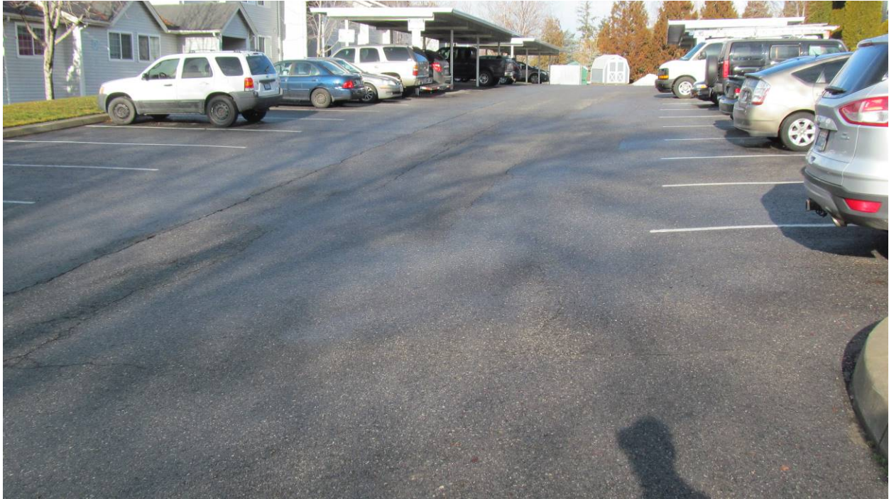
Photo 3: Paved Parking Area - from the northeast
