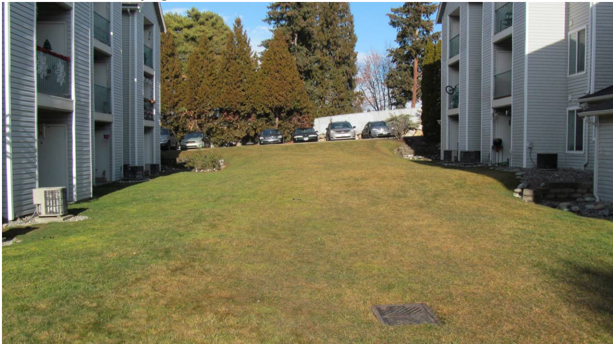
Photo 2: Site Landscaping - from the northwest
