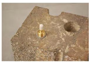
Figure 4. Installed Vapor Pin<sup>TM</sup>.
