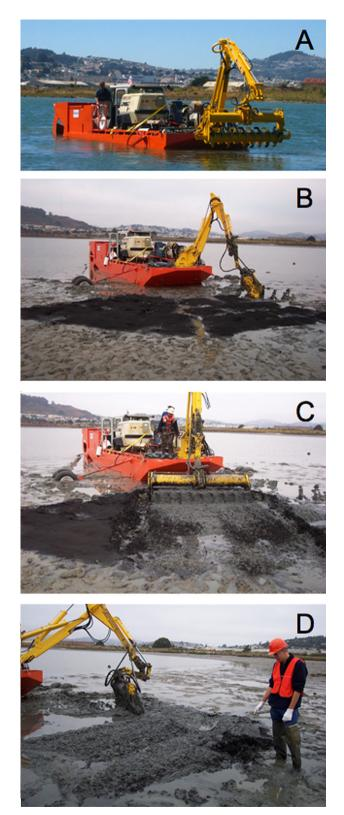
Fig. 2. (A) Mobilizing Aquamog to Plot A at high tide; (B) before, (C) during, and (D) after mixing activated carbon into sediment.
