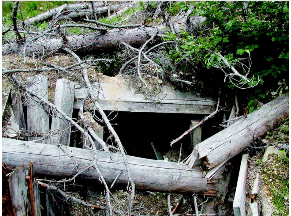
Figure 5. Collapsed portal of the St. Francis adit. View to the west.
