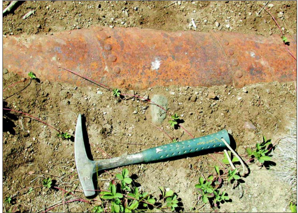
Figure 11. Riveted spirally constructed pipe carrying water from the powerhouse to the Chiwawa River. May be aqueduct outlet. Hammer for scale.
