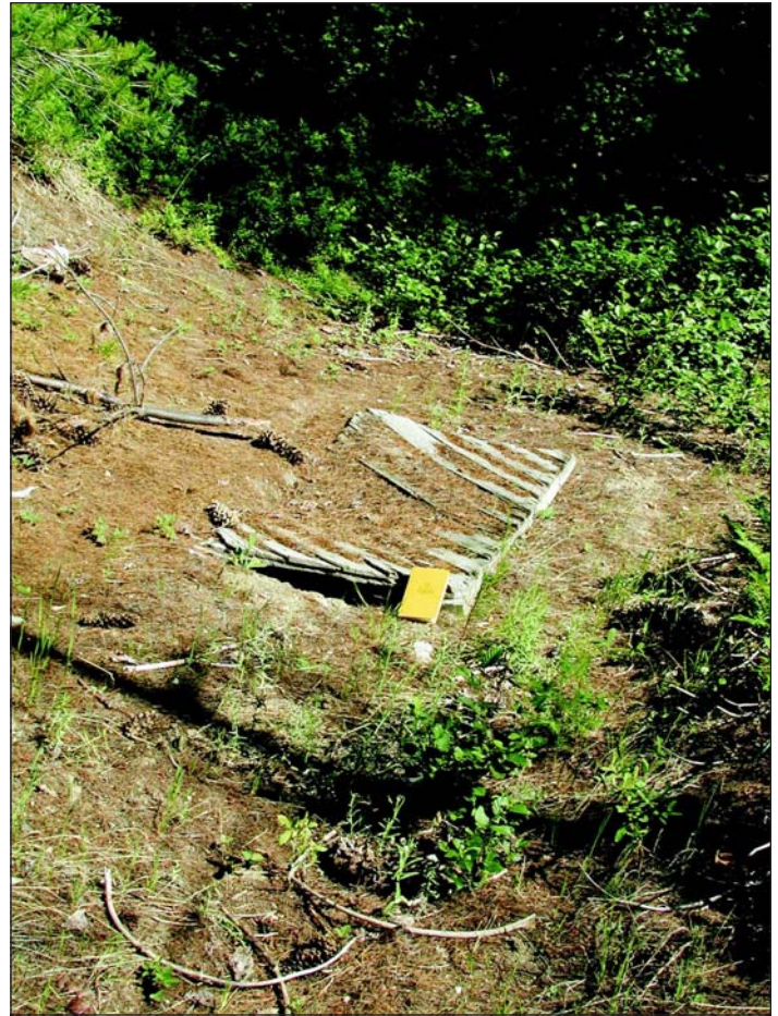
Figure 4. Deteriorating wooden covering over a hole near the banks of Chiwawa Creek. Notebook for scale.
