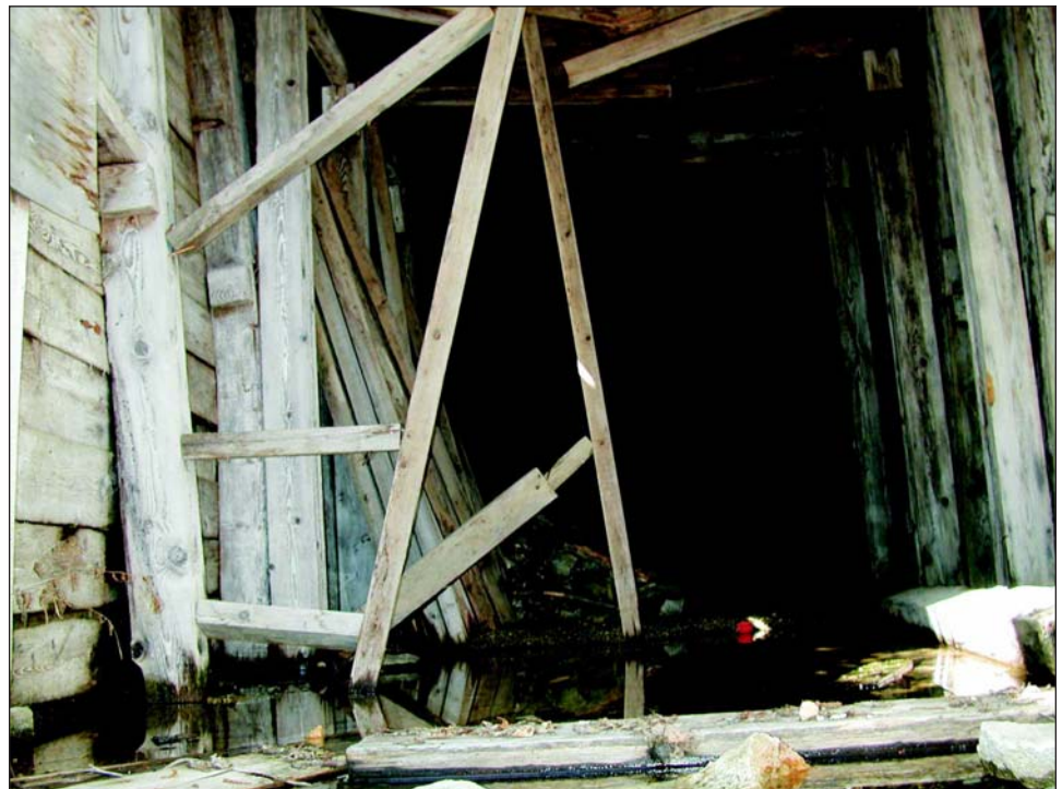
Figure 3. Trinity tunnel adit portal (bears N18°E). Photo taken through gap in wooden doors. Note sloughing inside on left.
