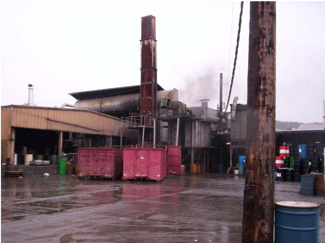
Photo 10: Industrial Container Services – smoke emissions from furnace
