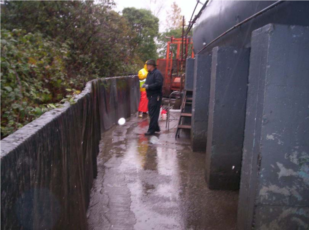
Photo 15: Area approximately 30 feet west of Well B-1
