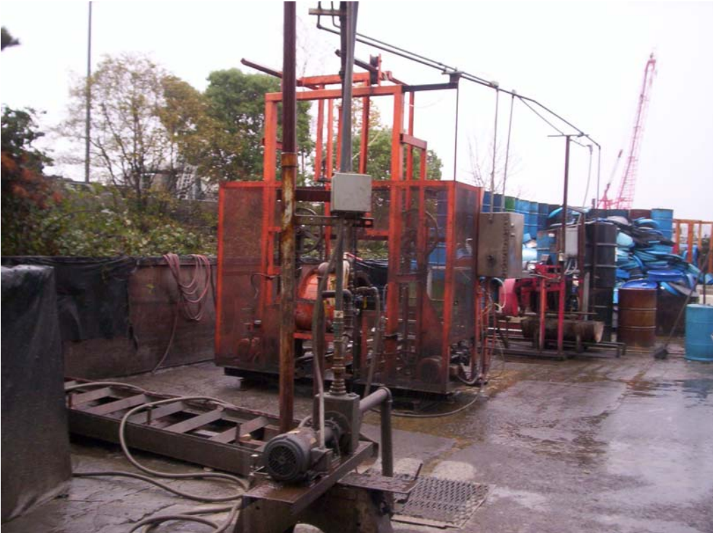
Photo 14: Looking east from Well B-1 along slip
