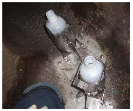
Figure 9. Sediment Traps Installed in a Storm Drain Line
