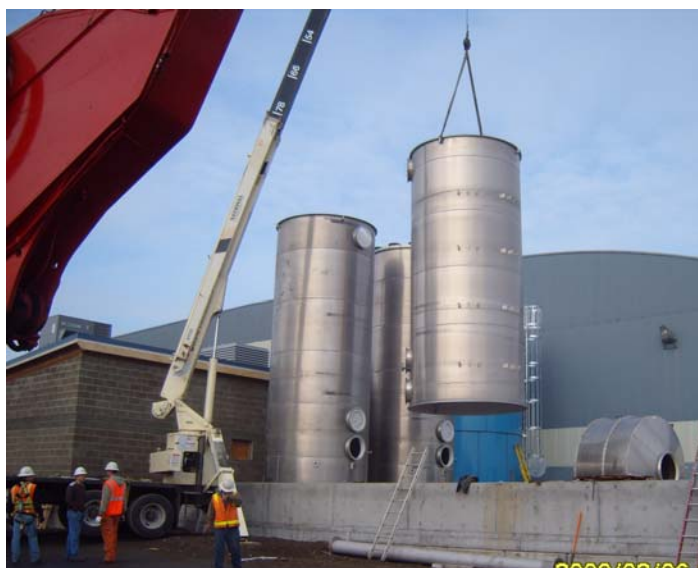
Installation of one of the air stripping towers.
