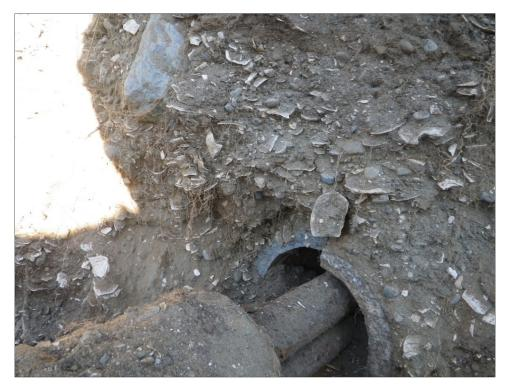
Figure 5-3. Shell layer within sand fill surrounding a concrete utility pipe found within the trench.
