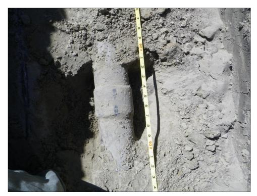
Figure 5-5. Overview of a joint in the westernmost fuel pipe.
