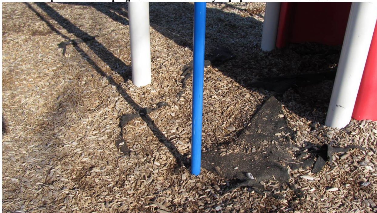
Photo 4: Exposed Landscaping Fabric Beneath Play Equipment – from the west
