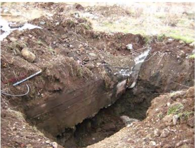
Figure 11. Concrete footer/foundation wall in TP-1.
