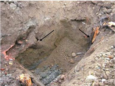
Figure 12. TP-6, showing wood stave pipe (left arrow) and piling (right arrow). Facing S.
