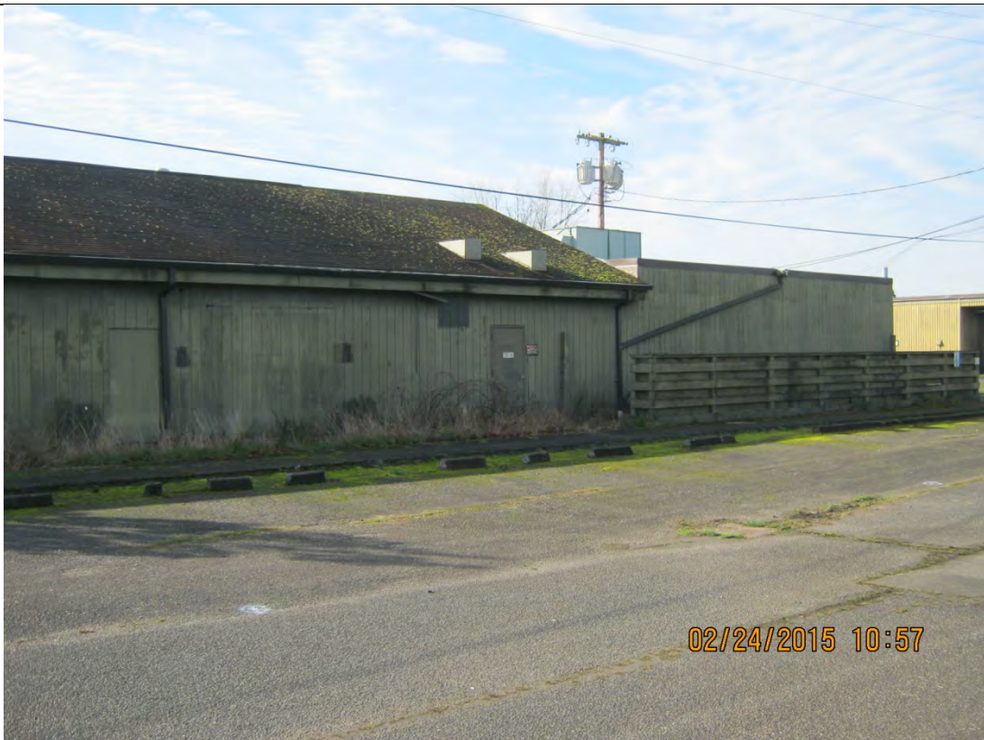
Photograph: 1 | 2008 underground storage tank removal area. View to southwest.
