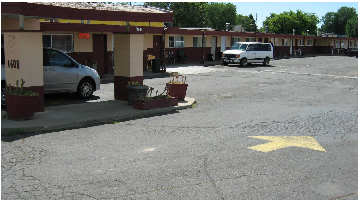
Photo 4: Inn Office and Rooms – from the northwest
