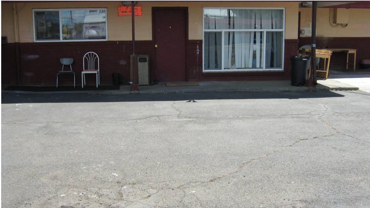
Photo 1: Former UST Location – from the west
