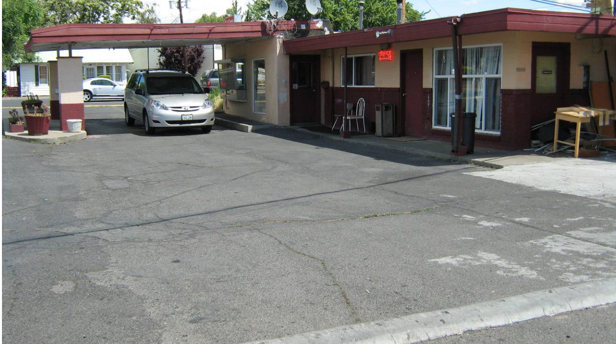
Photo 3: Office and Former UST Area – from the southwest
