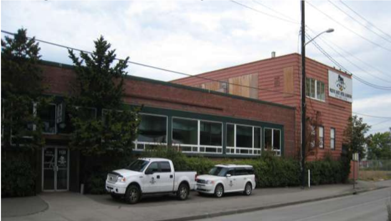
Photo 1: Spokane Street (south) side of building
