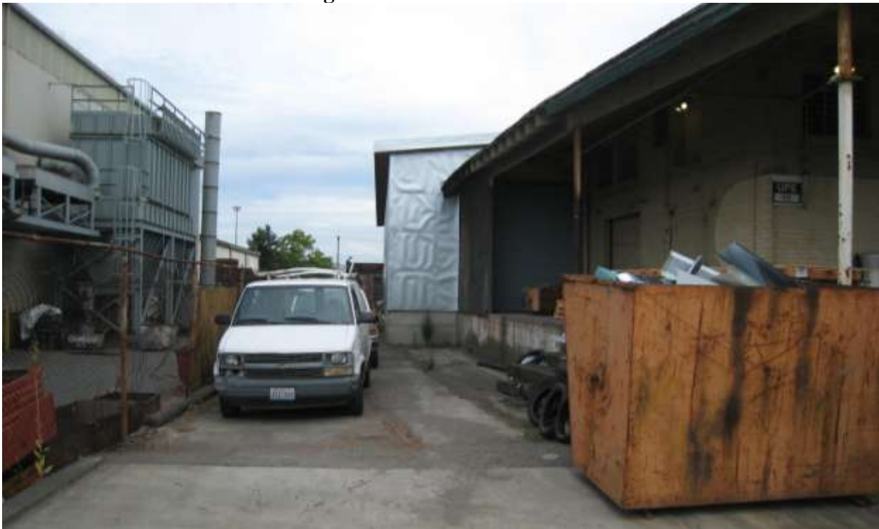
Photo 4: North side of the building – from the west
