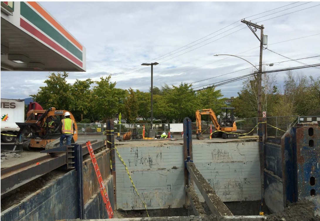
View of slide rail shoring
