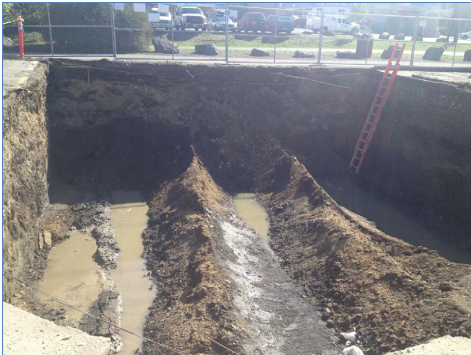
Picture looking east. Tank Basin following removal of three USTs
