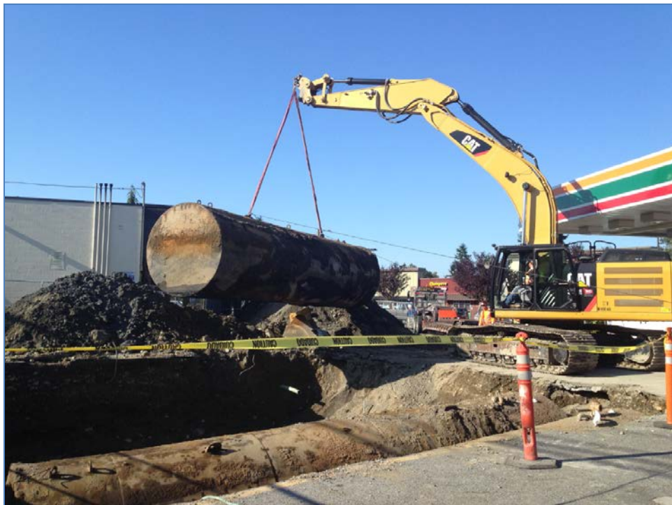
Removal of middle 12,000-gallon gasoline tank.
