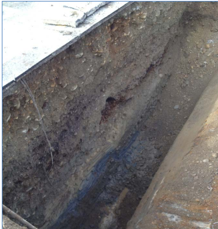
Picture looking northwest. View of western side wall.
