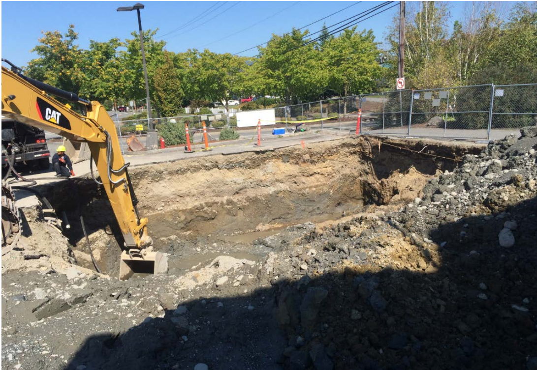
Remedial over-excavation
