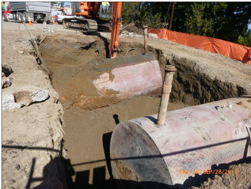
1. UST-1, UST-2, and UST-3 excavation and removal, looking north.
