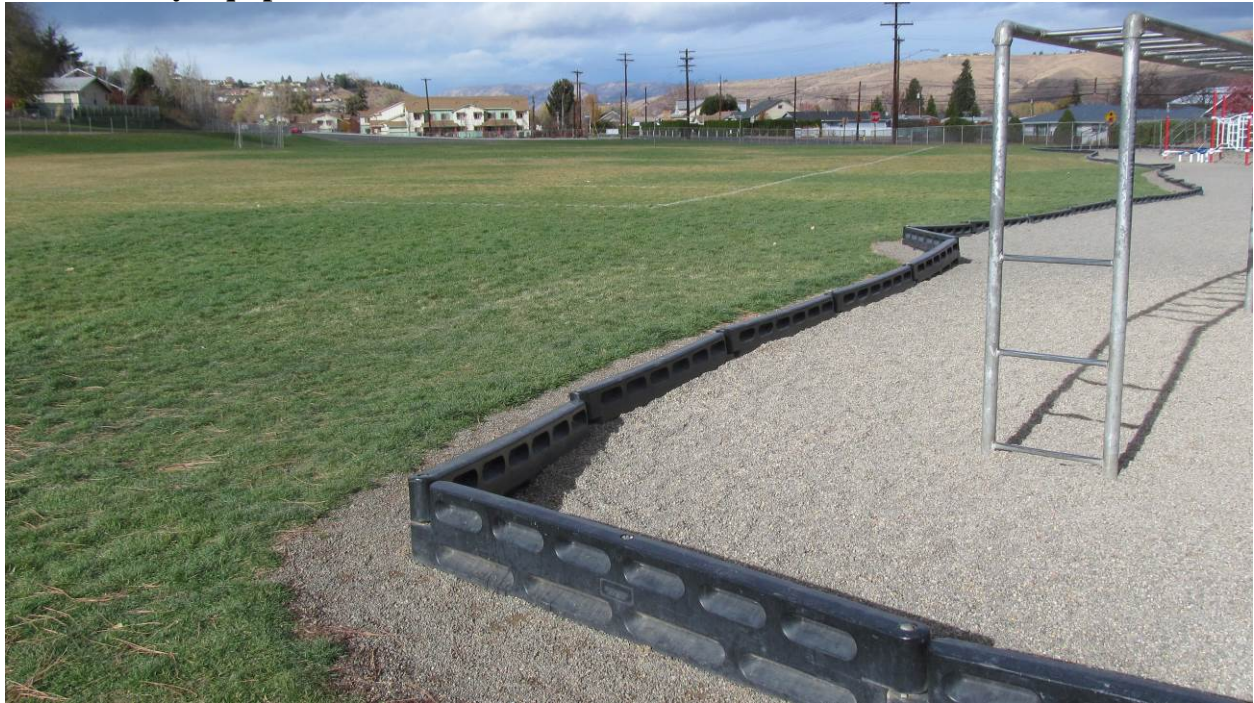
Photo 3: Play Equipment Borders and Pea Gravel Cover - from the south
