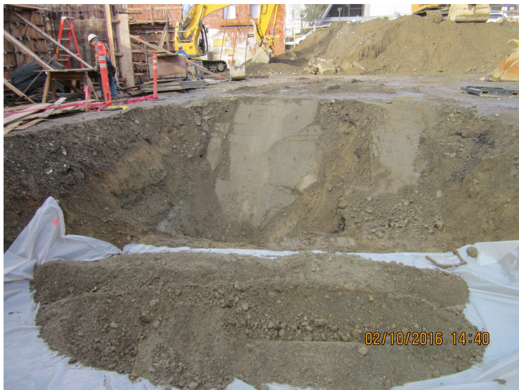
Photograph 10. Looking north at the excavation at the conclusion of removal activities with the stockpiled PCS in the foreground.
