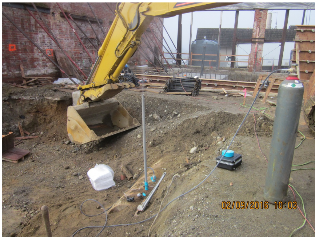
Photograph 4. S3 inerting the UST with carbon dioxide prior to removal.
