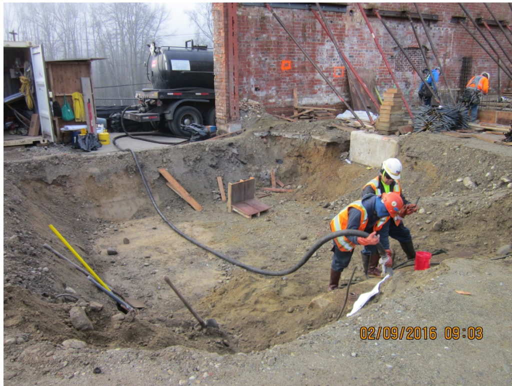
Photograph 3. MarVac triple rinsing the tank after removing the contents during decommissioning activities.
