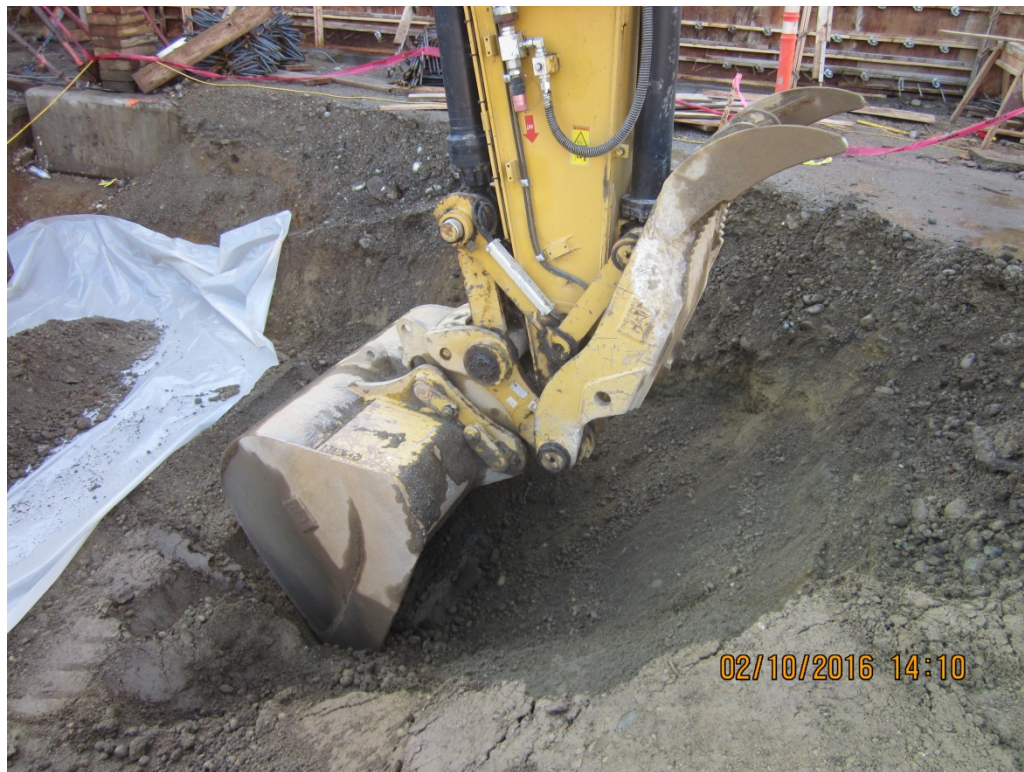
Photograph 9. Removing contaminated soil from below the former UST location, looking west.
