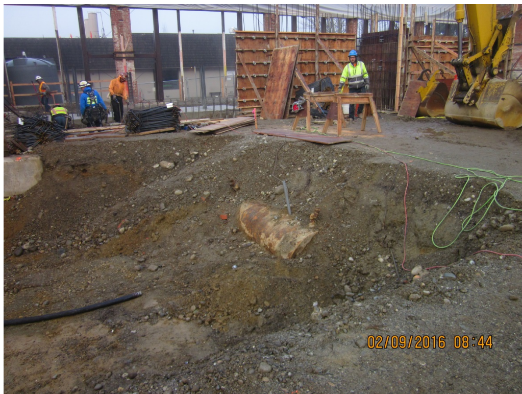
Photograph 2. Looking northwest at the UST prior to removal.
