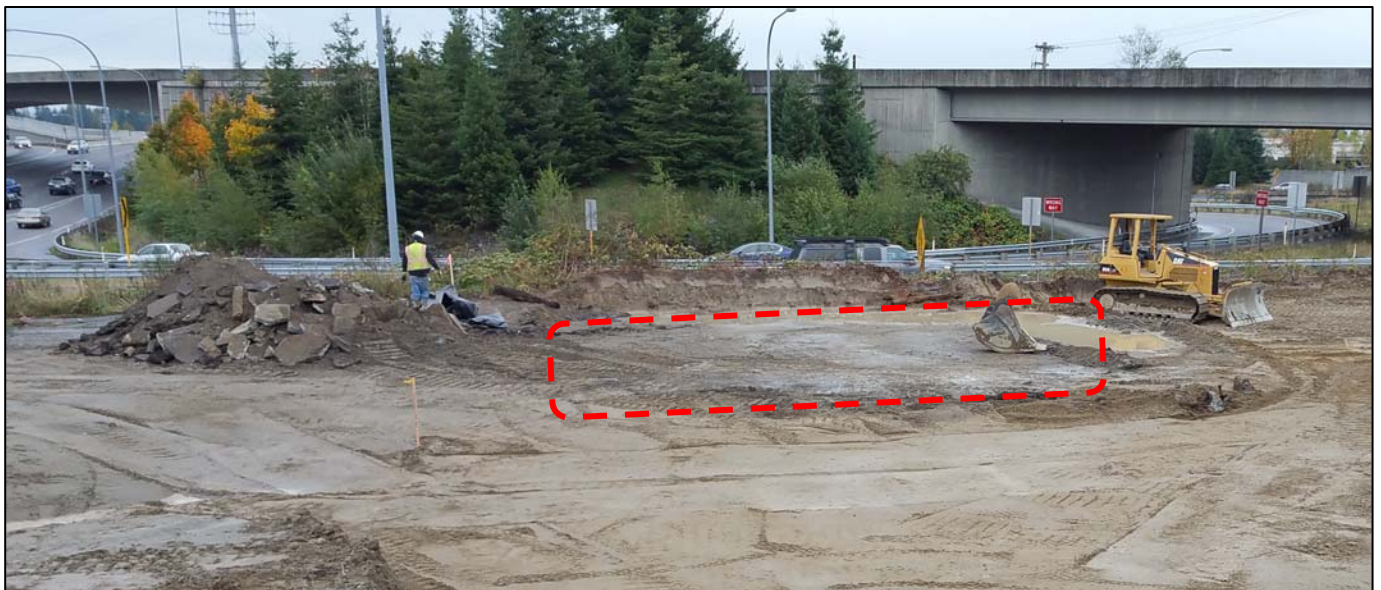
PHOTO B. Photo looking east shows area of concern on October 28, 2015 in red prior to excavation beginning. Upon completion an area approximately 36 feet long, 10 feet wide and approximately 3.5 feet deep at the ends becoming approximately 4.5 feet deep in the center.
