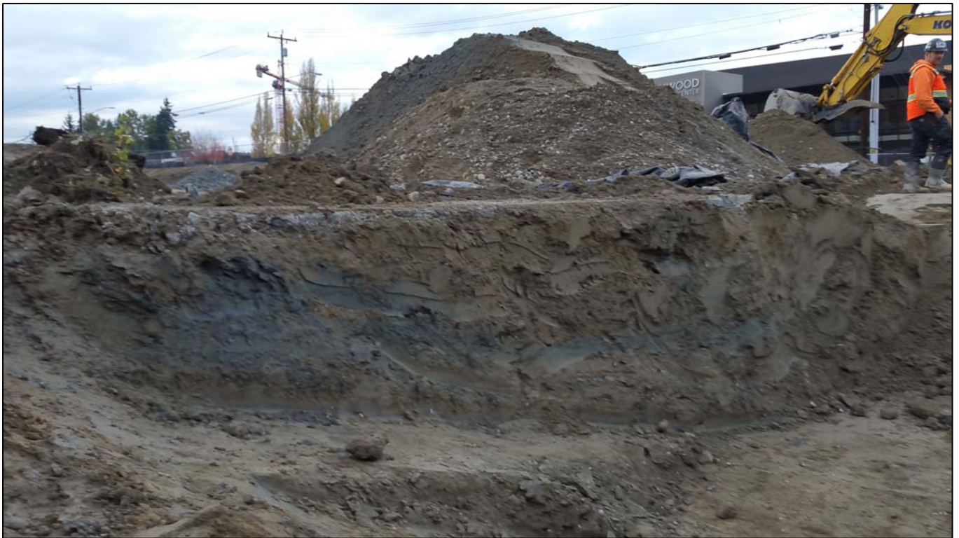
PHOTO D. Photo looking west shows area of concern during November 5, 2016 site visit where a vein of potentially contaminated soils was exposed in a trench along the east property boundary.
