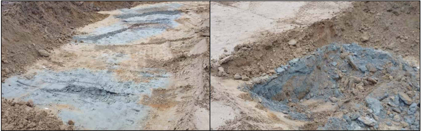
PHOTO C. Image on the left reveals potentially contaminated soils at the excavation of Set-2. Image on the right shows the north end of the excavation during removal. Note the difference in color between the suspected affected soils and their surroundings to sides and below.
