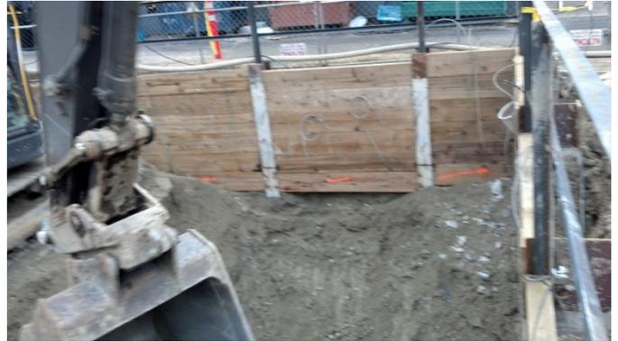
Subsequent UST soil excavation area after shoring installation
