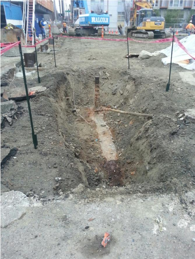
2,750 gallon UST exposed for cleaning and inerting
