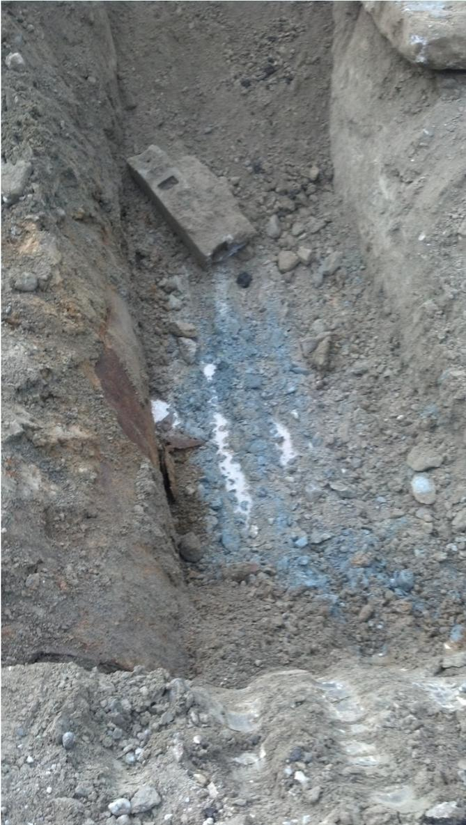
Soils adjacent to 2,750 gallon UST exposed for removal
