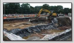
In areas A1 and A2, the plan is to remove contaminated material from the site and transport the material to a treatment or disposal facility.
