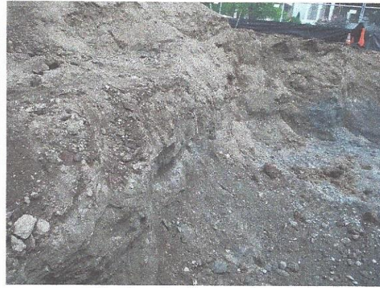
North wall of excavation pit
