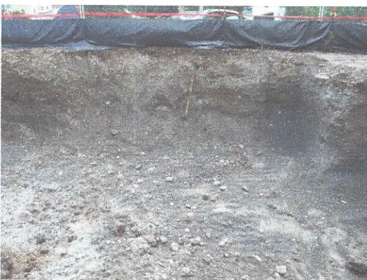
South wall of excavation pit
