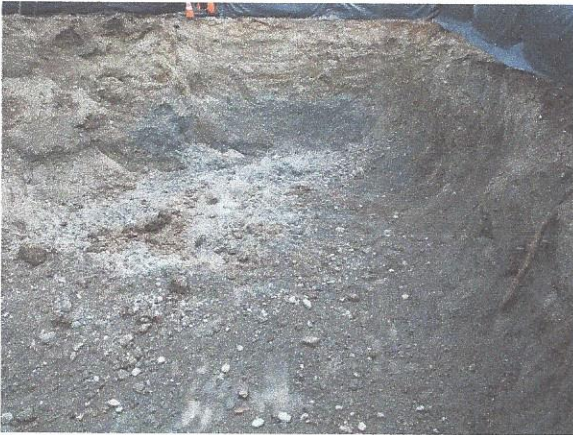
East wall of excavation pit
