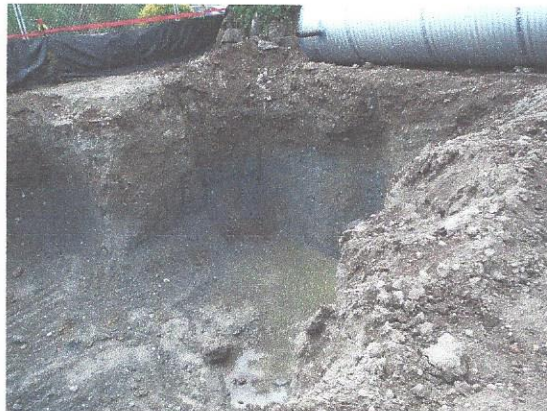
West wall of excavation pit
