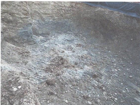
East wall of excavation pit
