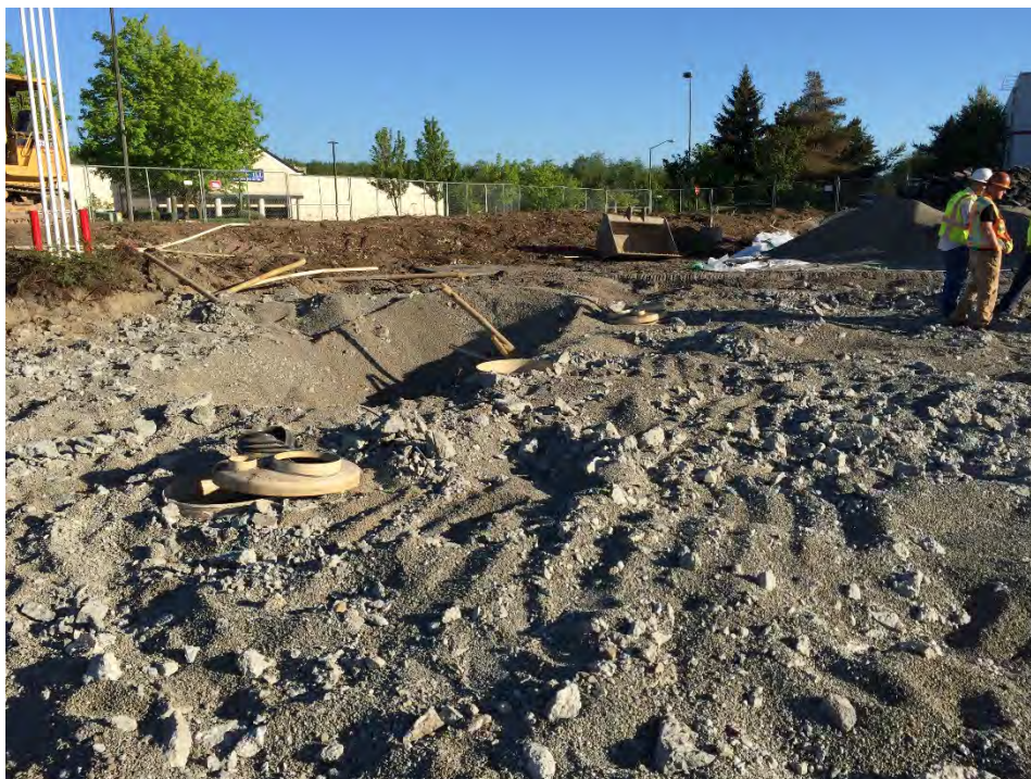
Photograph 2: View of exposed surface of underground storage tanks (USTs) prior to excavation, facing north.
