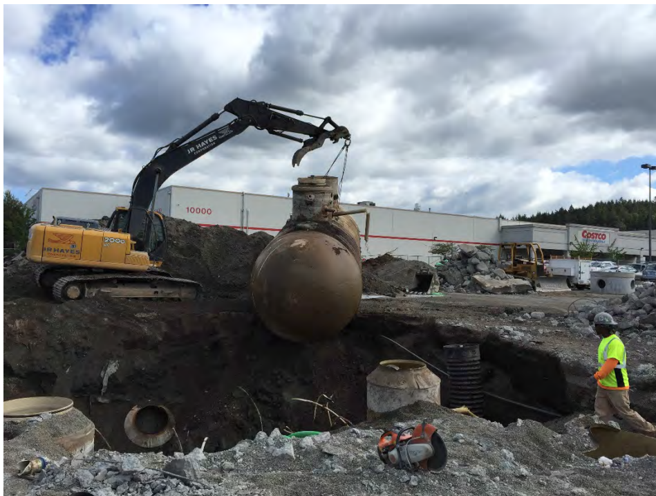
Photograph 3: View of UST #3 removal, the northmost UST, facing north.
