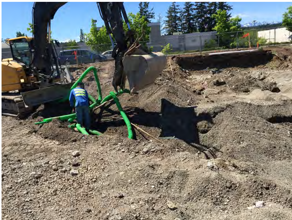
Photograph 8: View of product piping line removal between USTs and dispensers, facing west.
