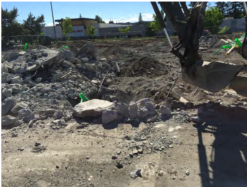
Photograph 9: View of removal of product piping lines and dispenser excavation, facing west
