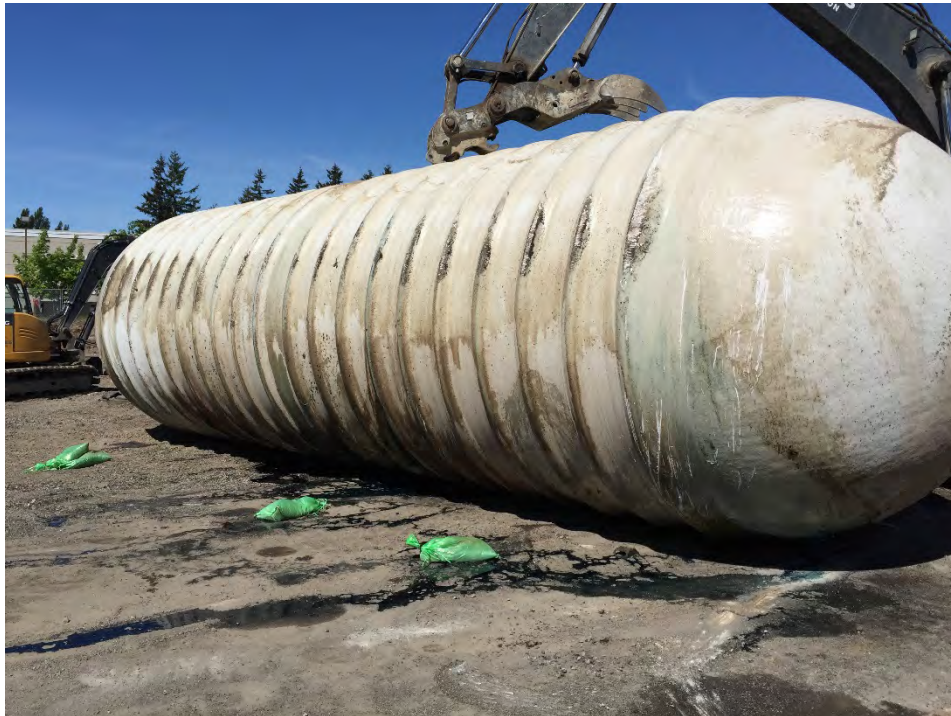
Photograph 7: View of on-site demolition of UST #1, facing northwest.
