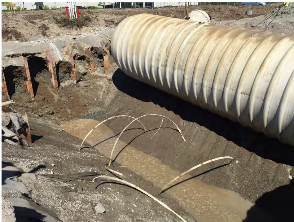
Photograph 6: View of UST #1 removal, facing northwest.
