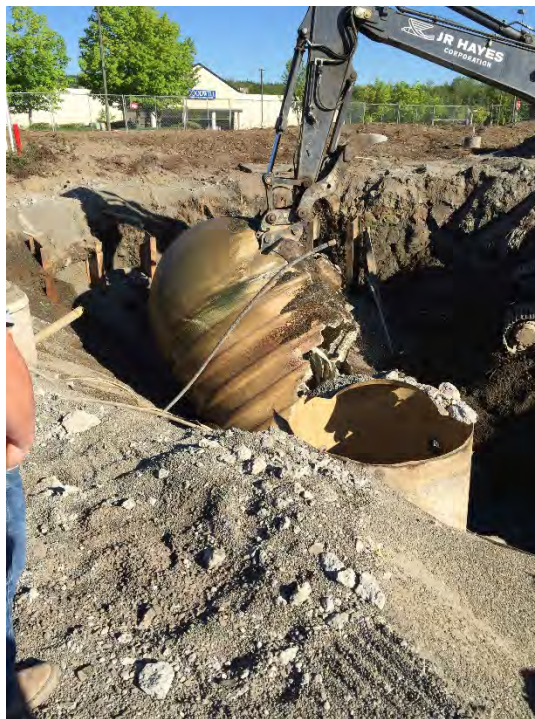
Photograph 5: View of in-place demolition of UST #2, facing northwest.
