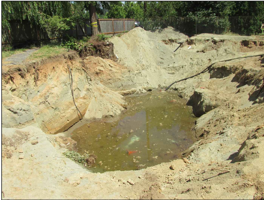
Photograph 9: View of remedial excavation just prior to excavation dewatering effort on July 20, 2016. No visible petroleum hydrocarbon sheen visible during this, or subsequent dewatering events.
