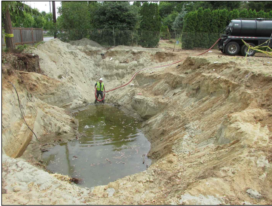
Photograph 11: View of remedial excavation just prior to excavation dewatering effort on August 2, 2016.
