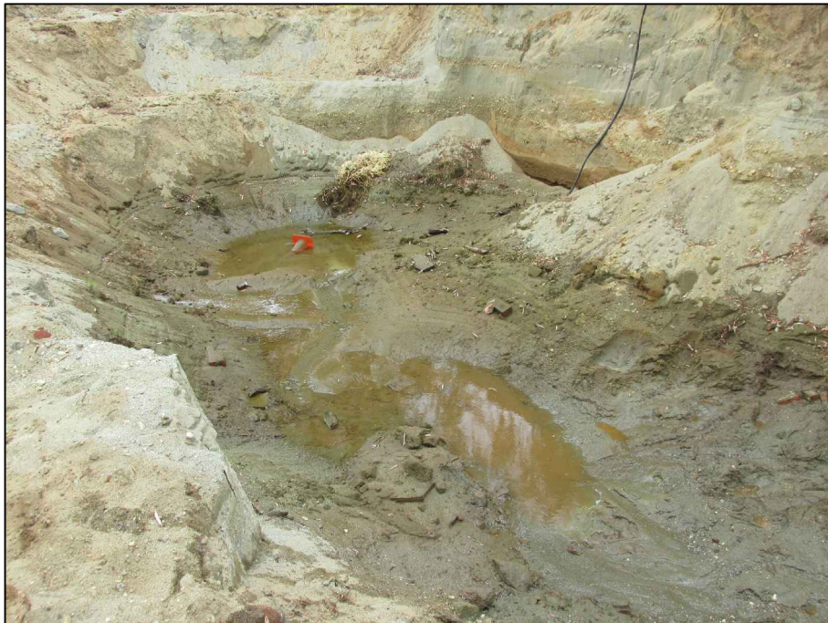
Photograph 12: View of remedial excavation following excavation dewatering effort on August 2, 2016.
