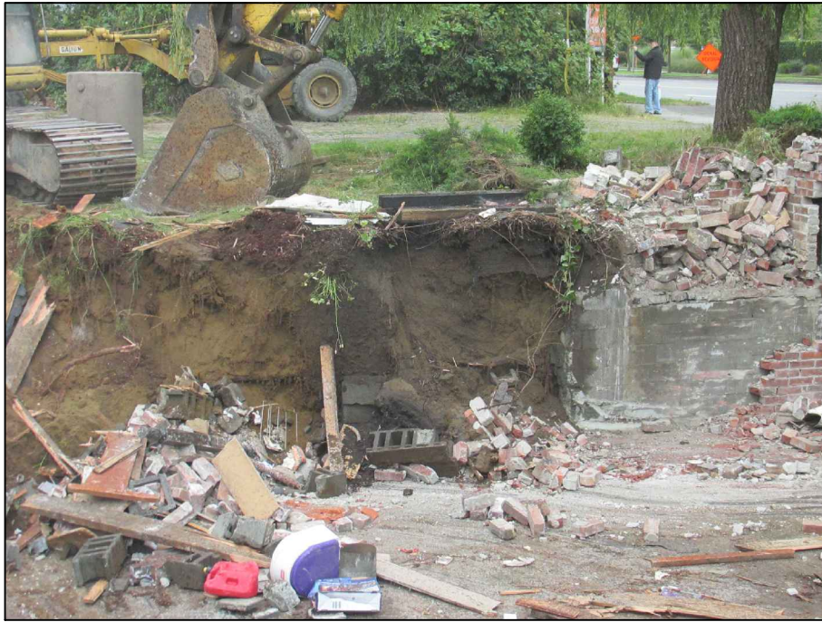
Photograph 3: View looking west at the basement's west wall during removal. Possible backfilled excavation (darker brown backfilled soils) visible just to the left (south) of chimney.
