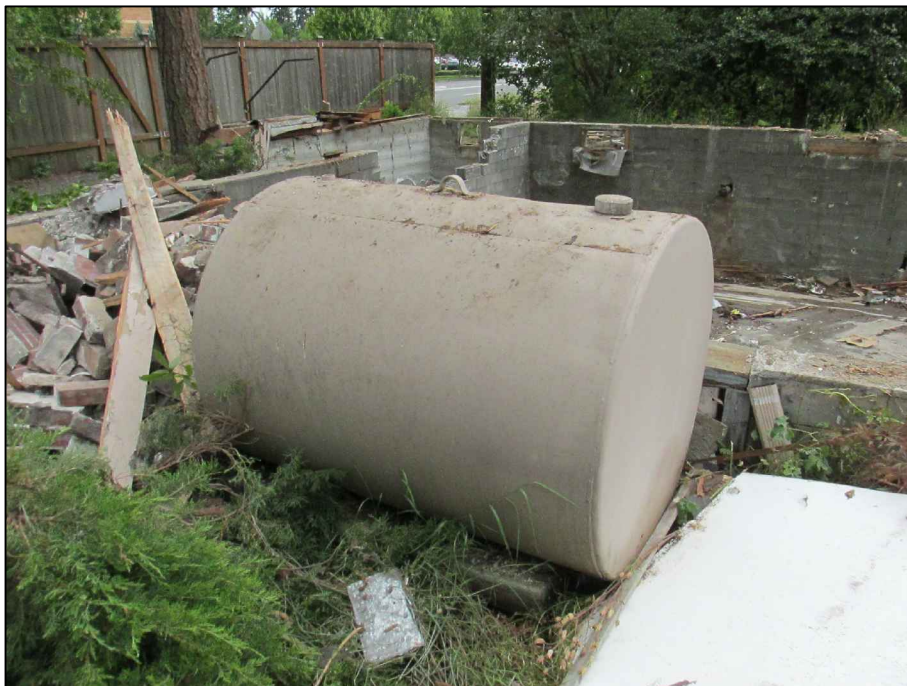
Photograph 4: View of heating oil AST in original location on the western side of former residence.
