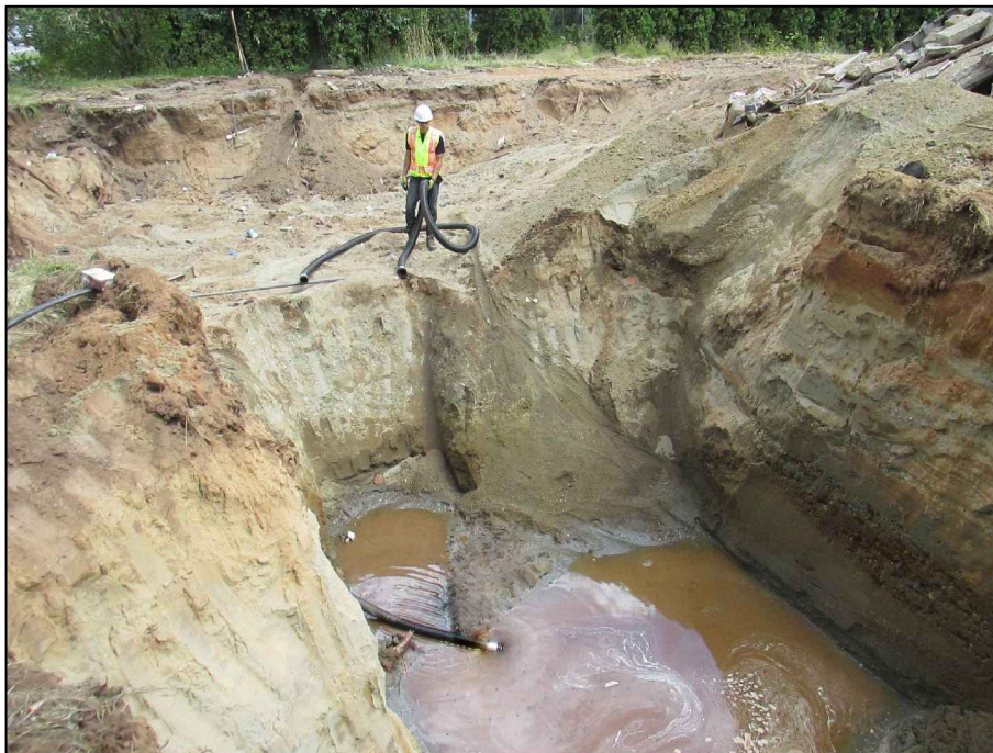
Photograph 6: View of remedial excavation limits (as of July 12, 2016) and excavation dewatering effort. Petroleum hydrocarbon (heating oil) sheen visible in photograph.
