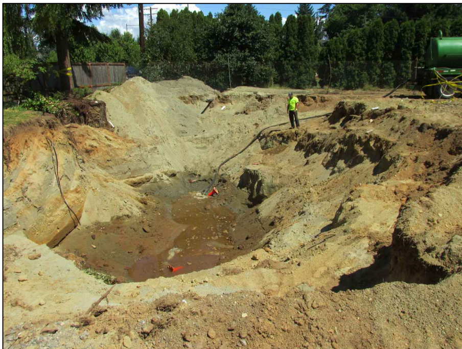
Photograph 10: View of remedial excavation following excavation dewatering effort on July 20, 2016.
