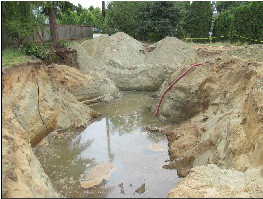
Photograph 7: View of remedial excavation just prior to excavation dewatering effort on July 15, 2016.
