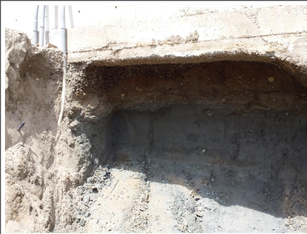
10. A total of five feet was excavated beneath Building H in order to verify that contaminated soils had been removed.
