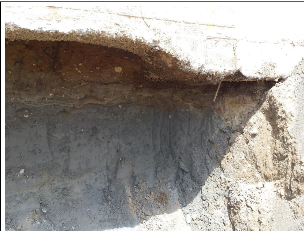
9. Excavation proceeded beneath Building H until it was determined that contamination was either very low in concentration or not present.
