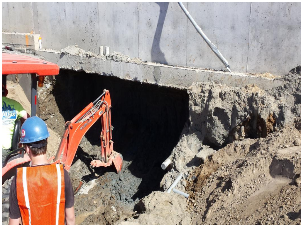
8. Following approval of undermining by structural and geotechnical engineers, contaminated soils were removed from beneath Building H.
