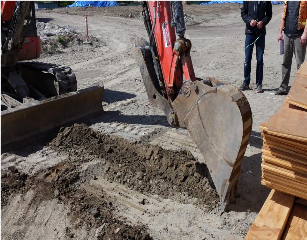
1. Initial excavation for characterization began in the eastern portion of the Grow Community Phase III site. Covered piles of contaminated soils can be seen in the background.
