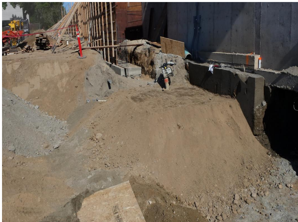
7. The western portion of the site was excavated beyond what appeared to be the margins of the plume, to where contamination was no longer indicated or suspected.
