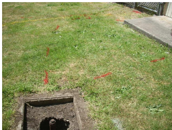
Photo #2: Location fill pipe and utility markings.
