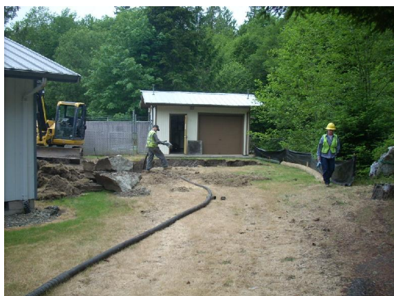
Photo #11: Excavation pit water removal.
