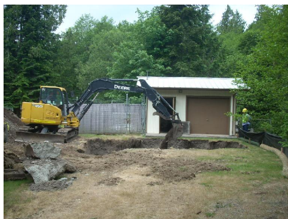
Photo #12: Backfilling.
