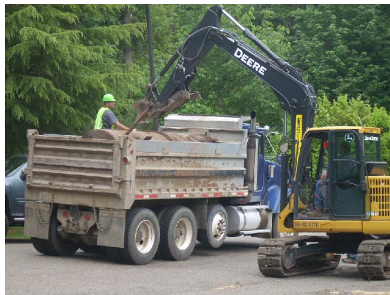
Photo #8: Underground storage tank being loaded for transport.
