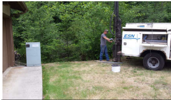
Photo #2: Boring #1 with former generator shed to the left of photo. ESN 5-10 feet bgs.
