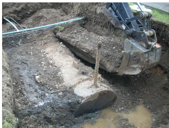
Photo #6: One of the UST's two concrete anchors.
