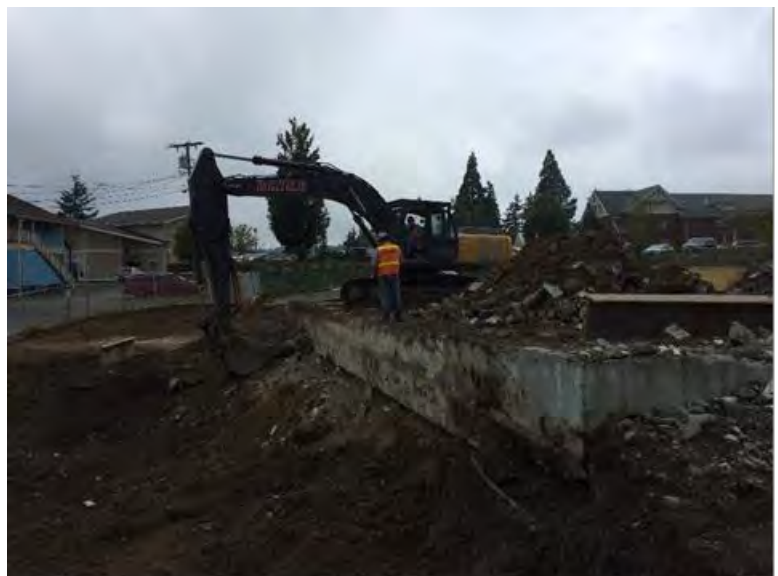
Photograph 3 - Building Demolition Exposes Soil to 12 feet in Some Locations of the Property
