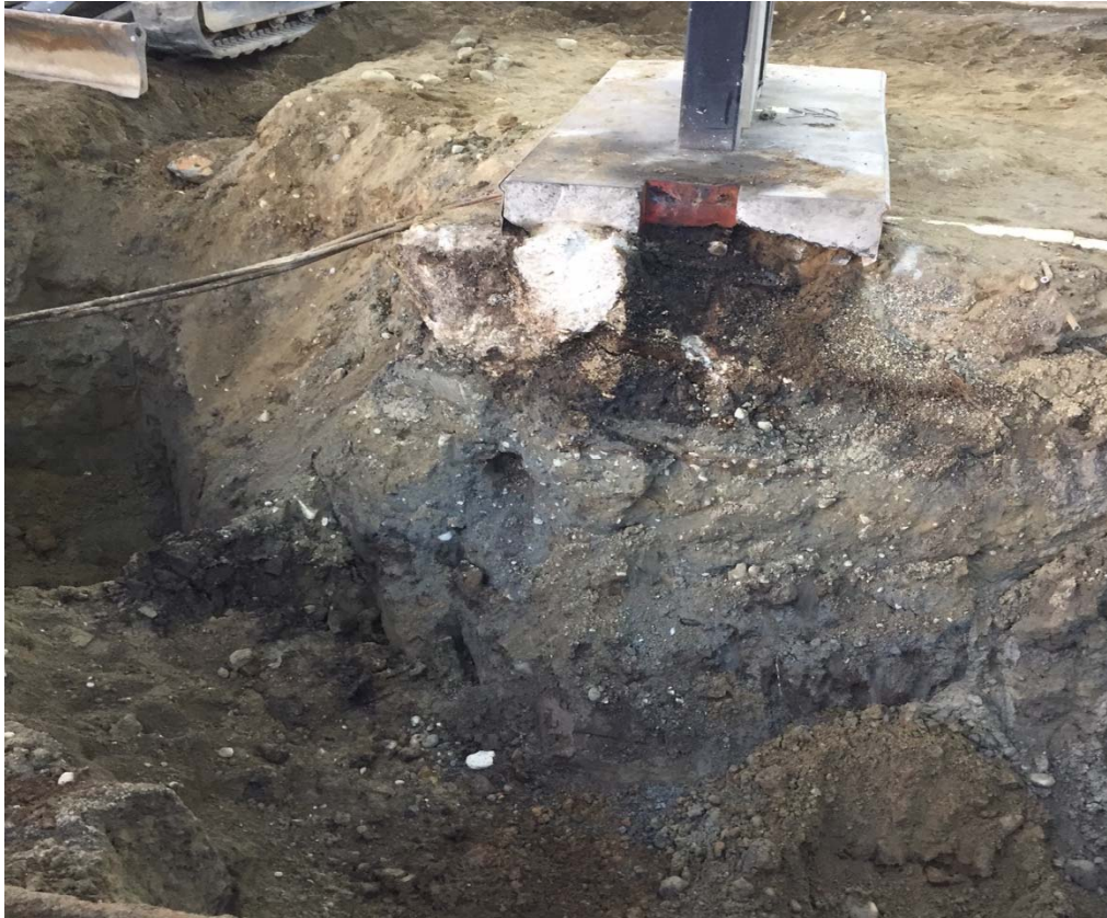
Photo 5. Petroleum contaminated soil visually observed beneath dispenser island numbers 9/10's concrete footing (looking north).
