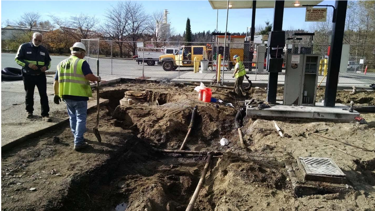
Photo 2. Initial exposure and evaluation of product piping south of dispenser island numbers 9/10 (looking west).
