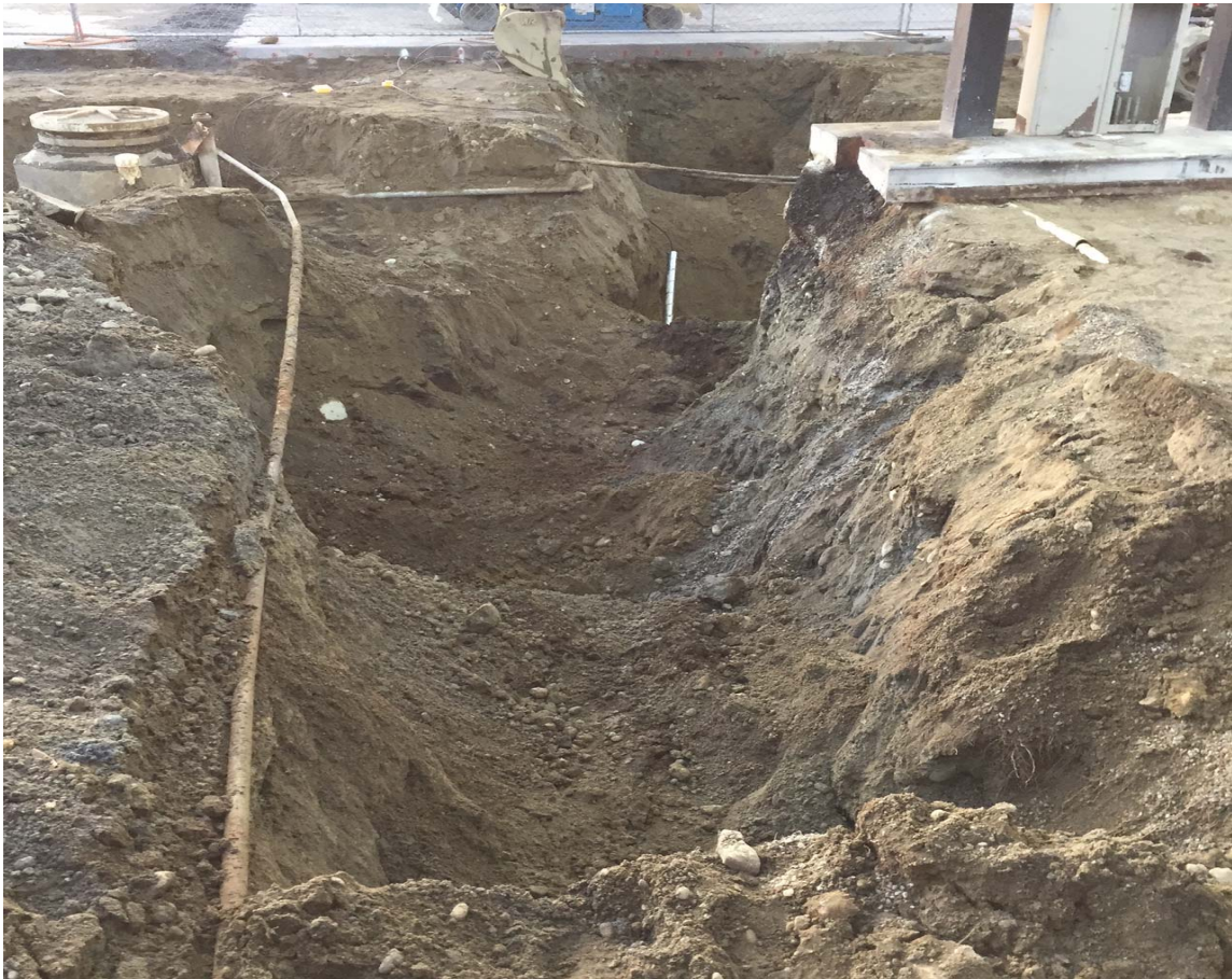
Photo 4. Petroleum contaminated soil excavation south of dispenser island numbers 9/10 (looking west).
