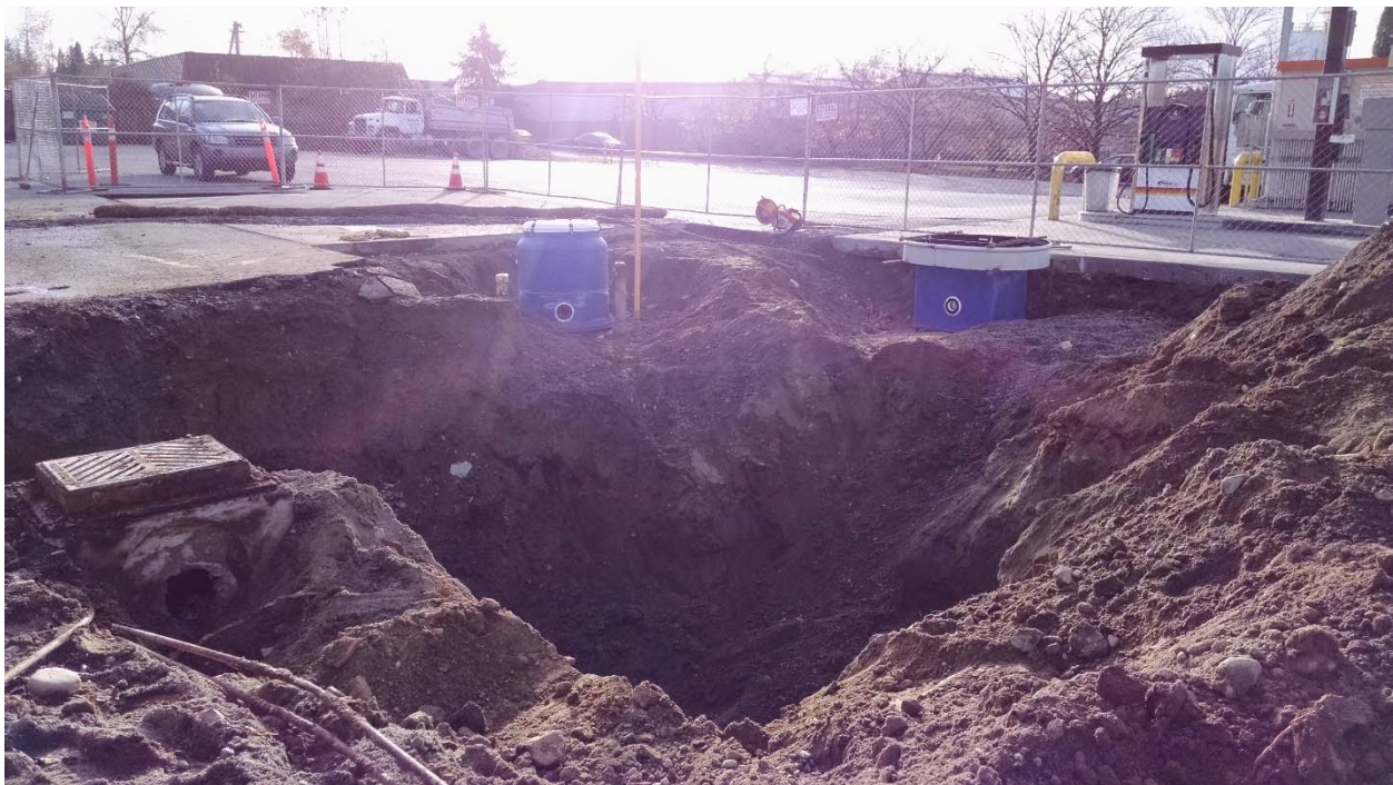
Photo 7. Over-excavation to remove additional petroleum contaminated soil associated with dispenser island numbers 9/10 and its concrete footing (looking southwest).
