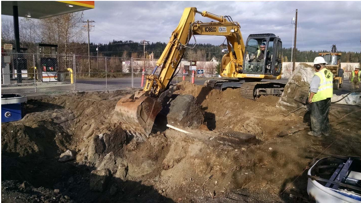
Photo 6. Removal of dispenser island numbers 9/10's concrete footing (looking south). Note: dispenser islands already removed.
