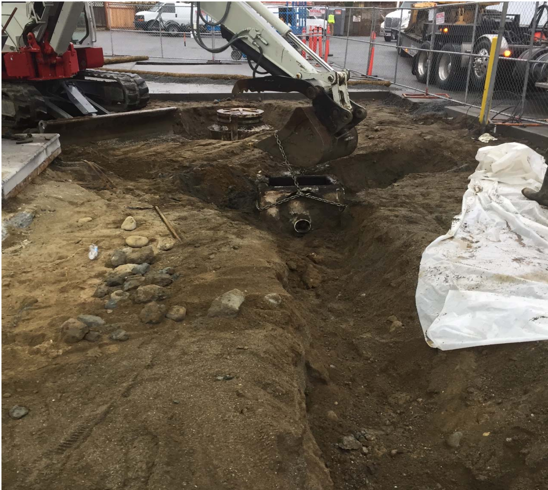
Photo 3. Removal of catch basin directly west of dispenser island numbers 9/10 (looking south).
