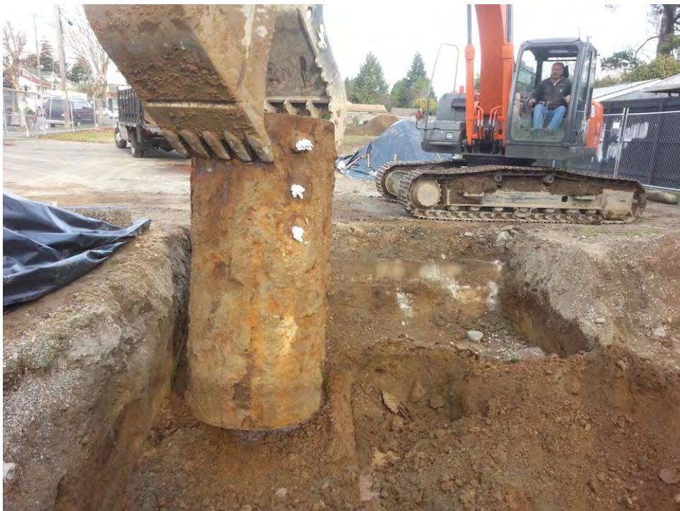
14.) View of Tank 3 after removal. The tank was in fair to good condition with moderate corrosion. (December 14 th , 2016)
