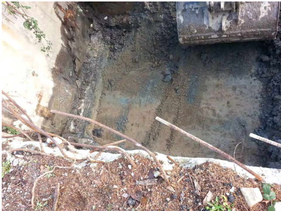
6.) View of clean soil in the excavation base, after removing about 1.5 foot of stained soil. (December 13, 2016)
