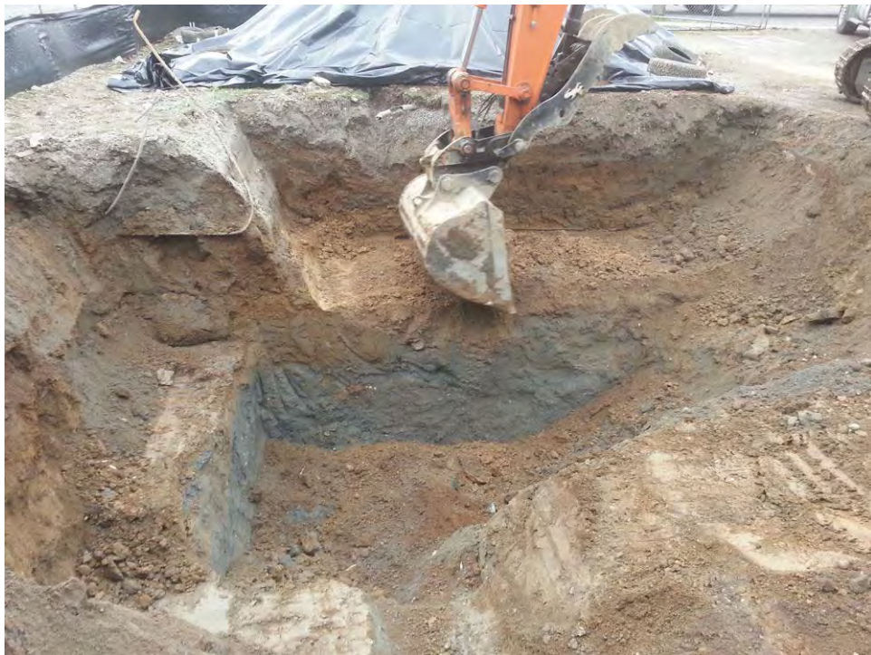
16.) View of excavation of petroleum contaminated soil. (December 15 th , 2016)
