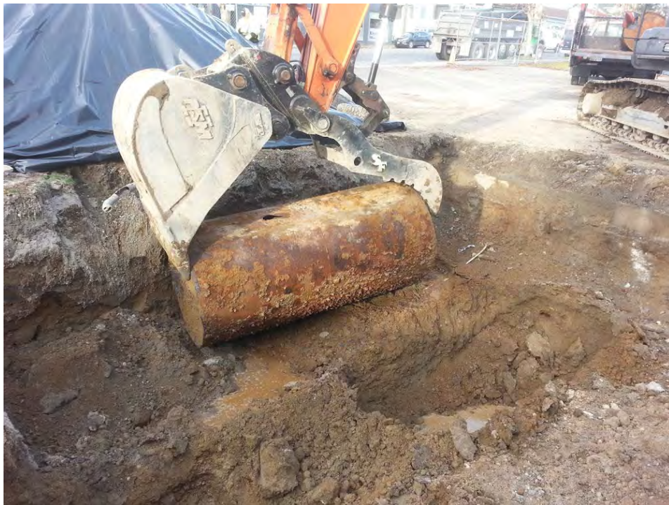
12.) View of Tank 1 after removal. The top of the tank had historically been partially cut open, but otherwise the tank was in good condition, with moderate corrosion. (December 14 th , 2016)
