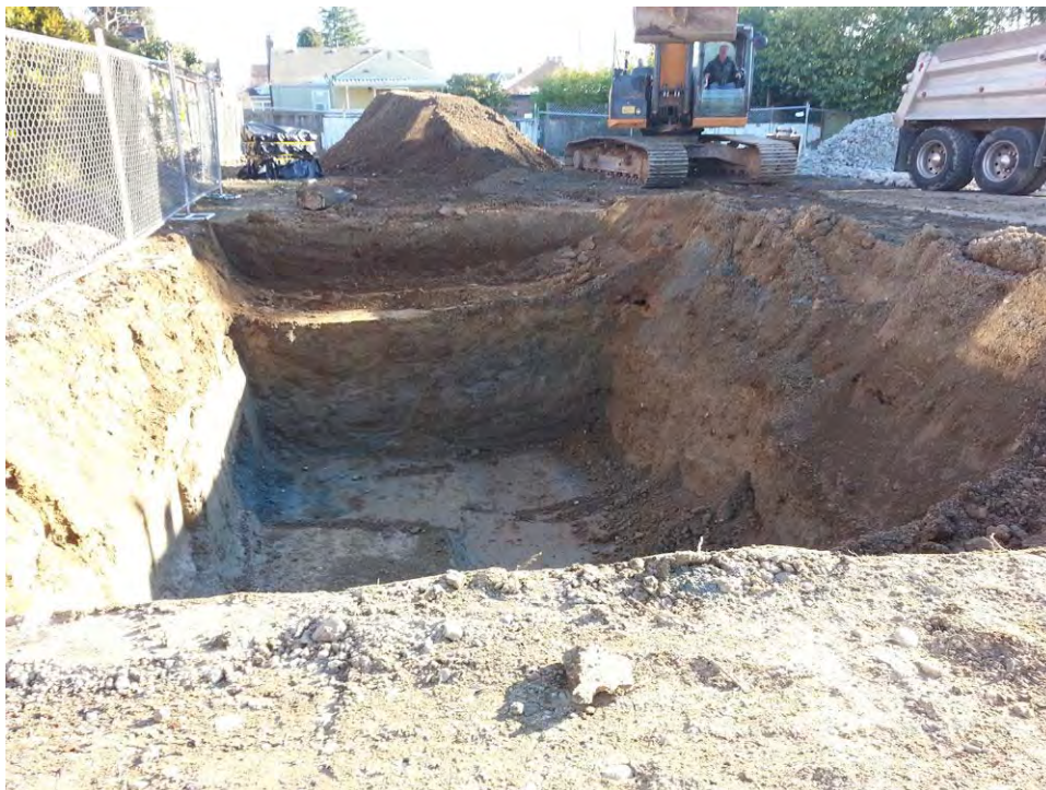
8.) View of the excavation of both lifts, nearing completion. A small zone of discolored soil remained at the north end of the eastern lift, on left. (January 3, 2017)
