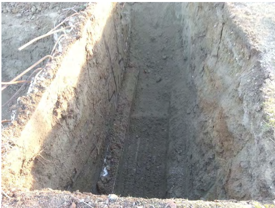
8.) View of the excavation outside the wall of the pit, to check if contaminants had seeped under the footing. West base sample taken from this area showed no detectable petroleum. (December 13 th , 2016)
