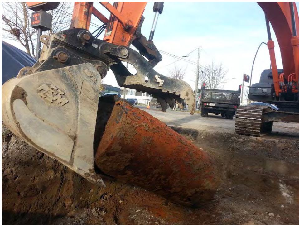
10.) View of Tank 2 after removal. The tank was heavily pitted, but there were no readily apparent holes. (December 14 th , 2016)
