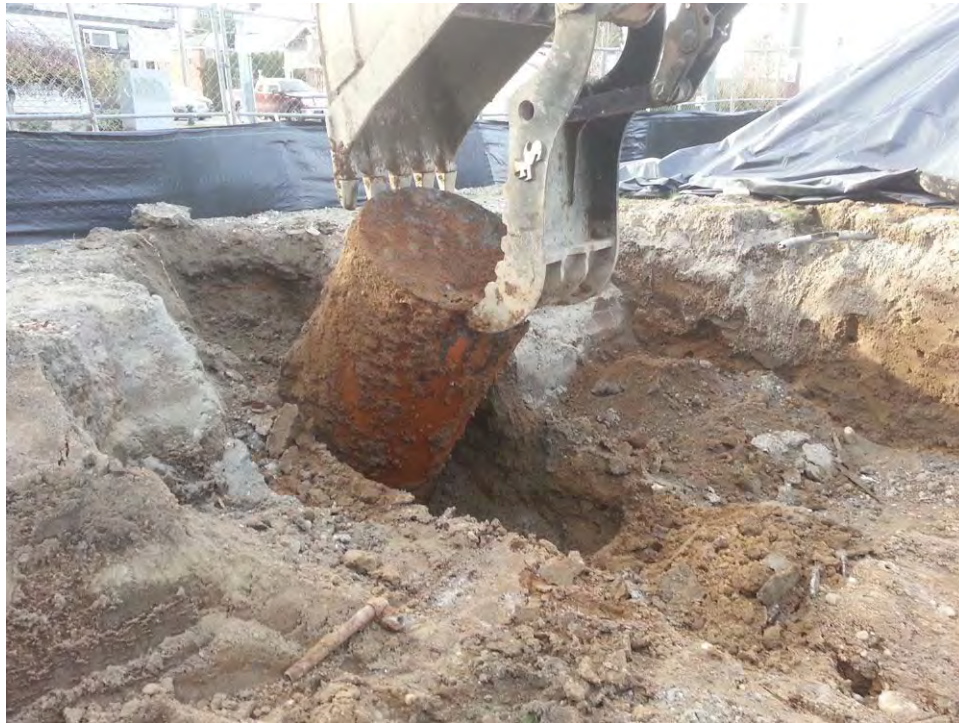
9.) View of Tank 2 being removed from the ground. (December 14 th , 2016)
