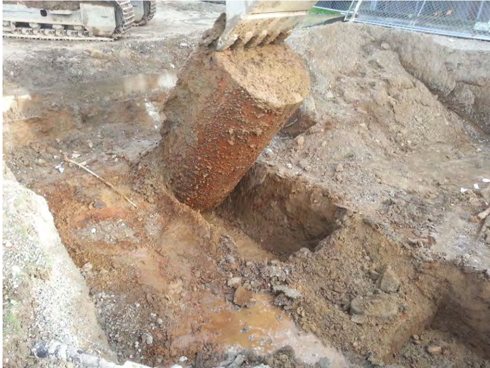
11.) View of the trackhoe removing Tank 1. (December 14 th , 2016)
