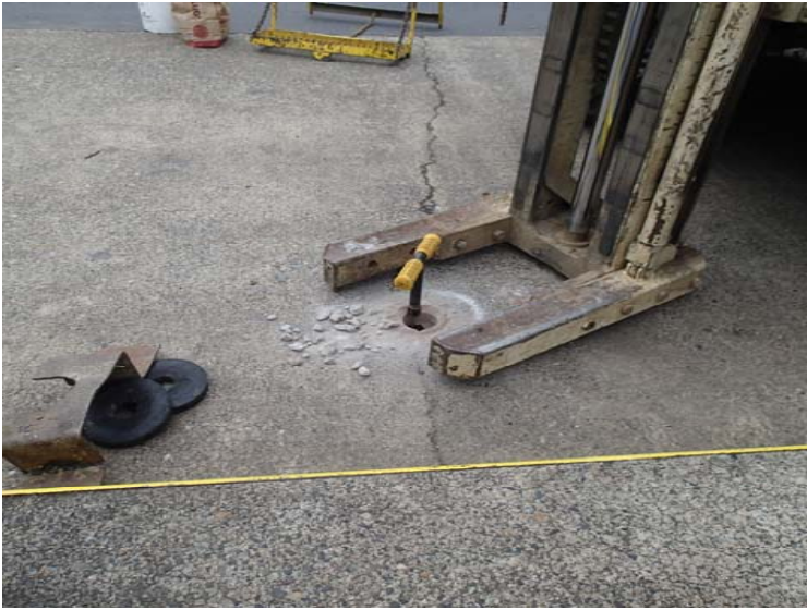
A 6-foot tile probe was used to manually clear holes prior to drilling to avoid damaging underground utilities near the existing tanks and pump island.
