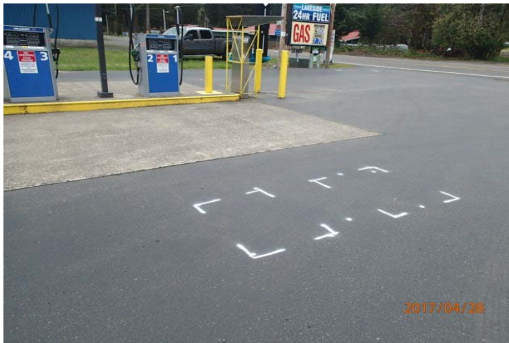
Magnetic anomalies were marked in white paint, and boring locations were sited in appropriate locations to assess suspect underground features.
