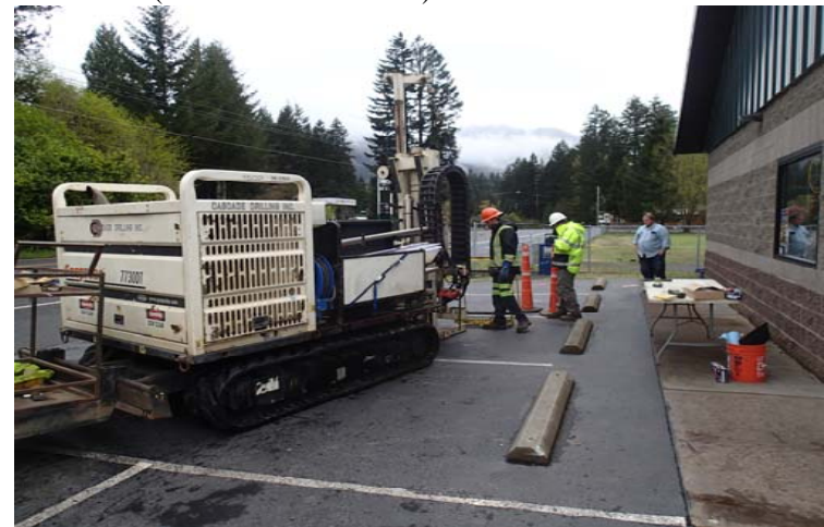
A GeoProbe drill rig was used to advance eight exploratory borings at selected locations.
