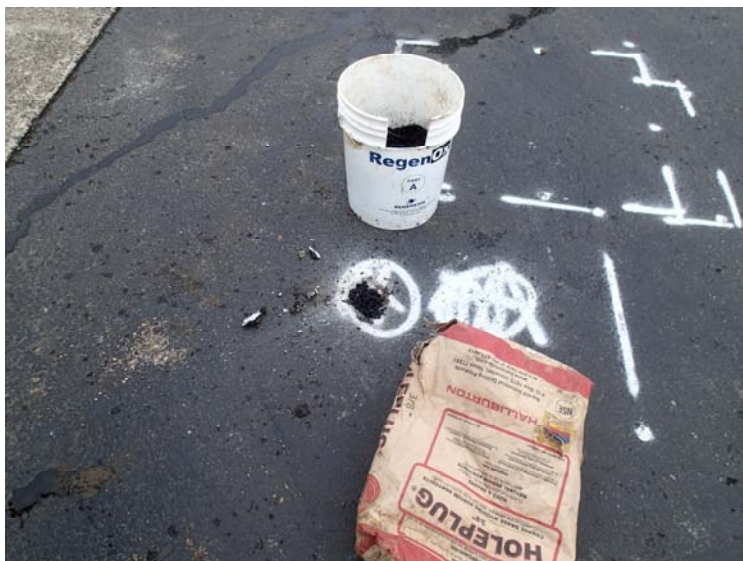
After drilling and sampling, each boring was backfilled with bentonite chips and sealed at the surface.
