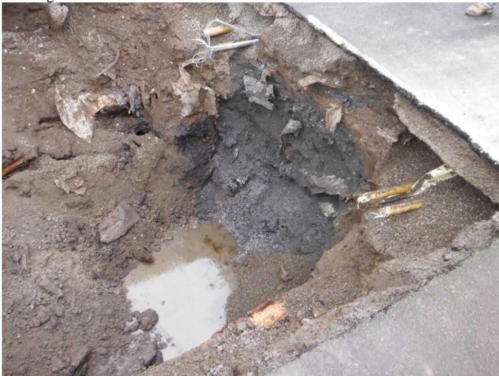
Visqueen barrier along north wall of tank pit, from removal of 3 adjacent USTs in 1989. Looking northwest.
