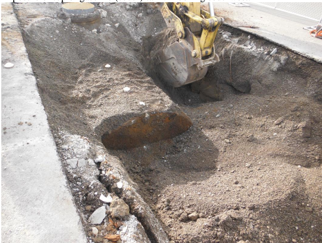
Exposure of top of gasoline (south) tank. Looking southwest.
