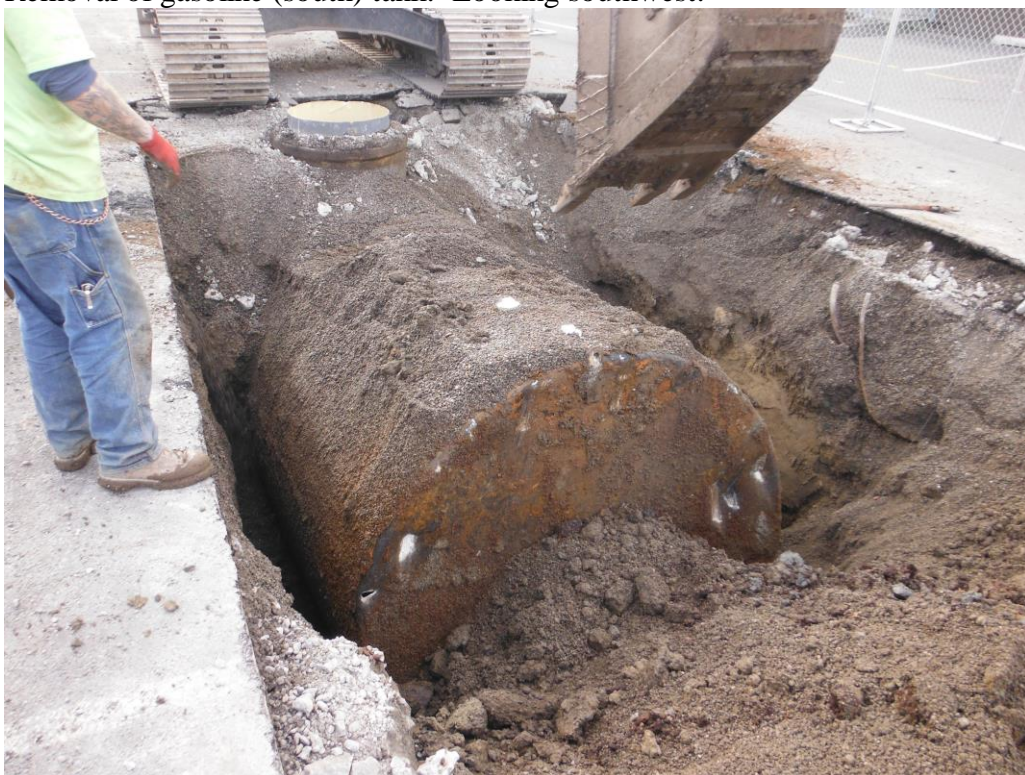
Removal of gasoline (south) tank. Looking southwest.
