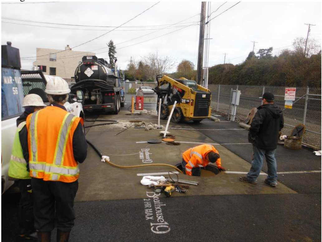
Removal of concrete pavement above the tanks. Looking north. Fuel dispenser in background.
