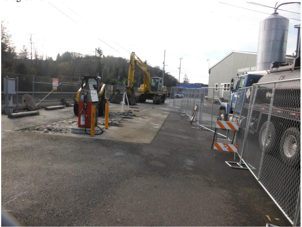
Removal of concrete pavement above the tanks. Looking south. Fuel dispenser in foreground.
