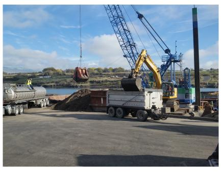
Loading stabilized sediments into trucks for trip up the hill to the landfill.
