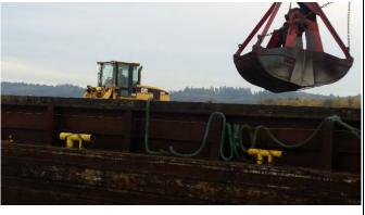
Comment: 10 CY Atlas cleanup bucke placing backfill sand.
