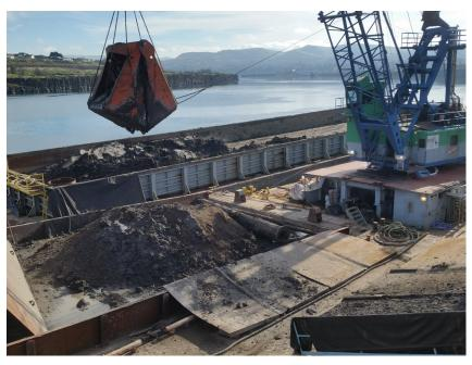
Offloading sediments from a haul barge to the sediment mixing bin. Note the spill plates and splash guards to contain any spillage.
