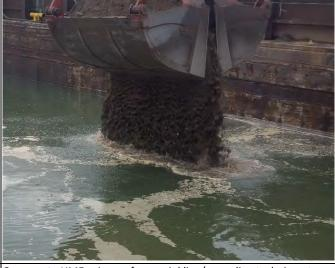
Comment: Offloading backfill material from clean fill Barge #31 and Comment: HME using surface sprinkling/spreading technique to placing on shoreward edge of dredge prism.
