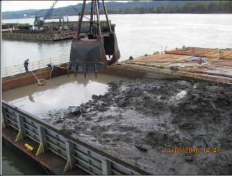
**Comment:** Barge nearly full and pumping free water from the barge into the water management barge.
