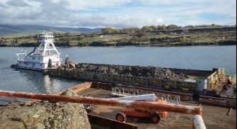
Comment: Pacific Power Vac. (sub to HME) 120 bbl vacuum tanker transferring water from tank on barge #BK5 for transport and disposal at Wasco County Landfill.
