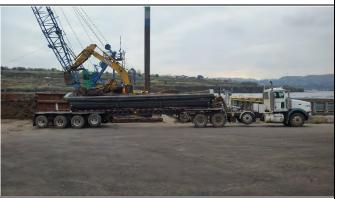
Comment: Oversized woody debris segregated on deck of barge #6 | Comment: Loading oversized woody debris to side dump trailer
