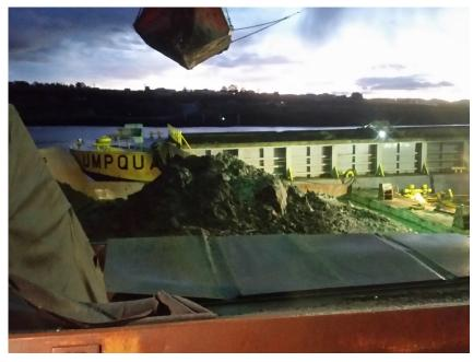
Offloading a haul barge at The Dalles, Oregon. Note the spill apron and fabric to prevent spillage into the river.
