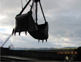
Comment: Placing sediments in Scow #6 with rehandling bucket.
