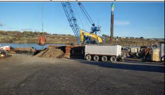
Comment: 120 bbl tanker removing water from tank on barge #BKS | Comment: Loading sediment to haul truck. for transport and disposal at Wasco County Landfill.
