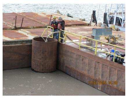
Dewatering free water off sediment haul barge to water management barge.
