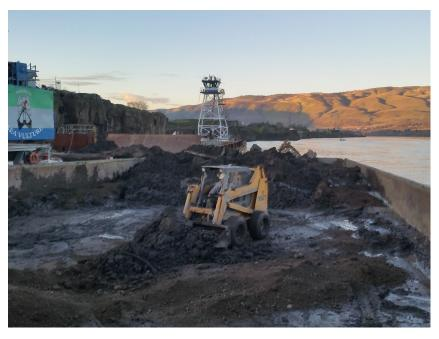
Stacking the last of the sediments on a haul barge to facilitate the removal by the clamshell bucket.
