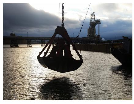
About to open the bucket to spread the backfill. Note the buoys that delineate the outfall's location.
