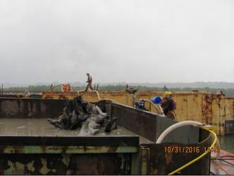
**Comment:** Large wood and root structures removed from site and crew addressing dewatering hoses to water management barge.
