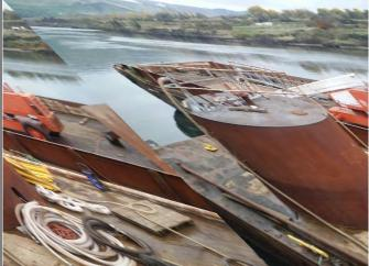
Comment: Installing drip plates between dock structure and Barge | Comment: Water storage tank positioned on Barge #BK5 #BK5
