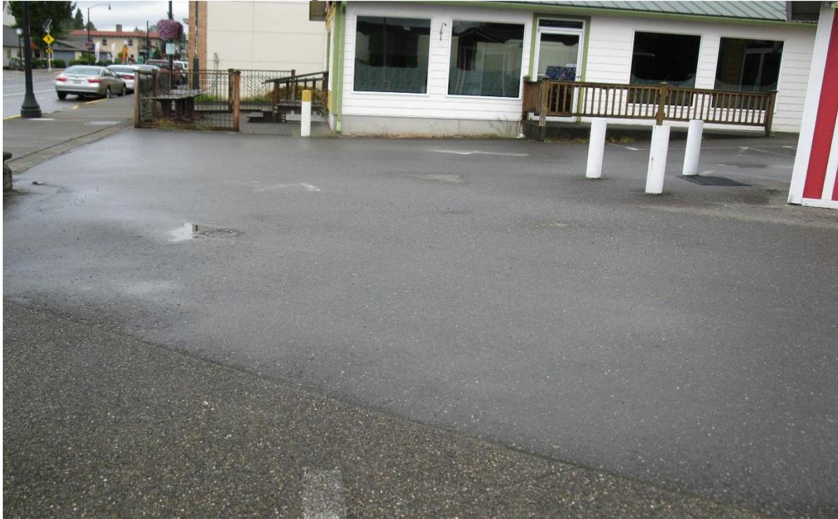
**Photo 4: Approximate Area of Contaminated Soils Left-in-Place at the Corner of 5<sup>th</sup> Street and the Alley and Asphalt Cap – from the Northeast**
