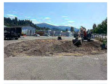
Photo #2. Removal of clean overburden fill soils.
