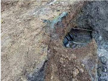
Photo #4. A 24-inch PVC storm water pipe was encountered along the west side of the remedial excavation. The pipe was not damaged by the excavator, instead water appeared to be leaking from a faulty pipe join.
