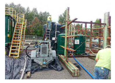
Photo #9. Dewatering effluent was treated with a sand filter and activated carbon, sampled and analyzed for TPH and BTEX, and discharged to the sanitary sewer under a King County permit.
