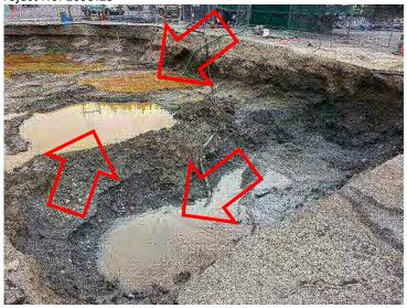
Photo #10. Rectangular-shaped areas that had been backfilled with pea gravel are assumed to be the former location of the three USTs removed in 1989.
