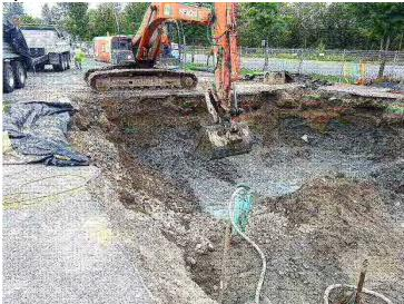
Photo #7. A sump was installed in the remedial excavation to extract water for treatment and subsequent permitted disposal to the King County sanitary sewer system.
