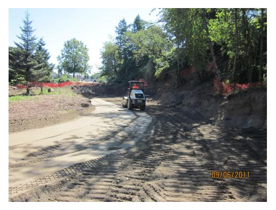
Photo 14. Compacting/rolling fill in Area 1.
