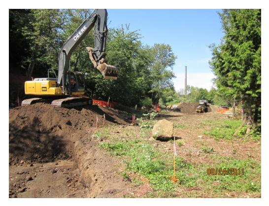
Photo 3. Excavation of Area 1, loading, and stockpiling within boundary of Site.
