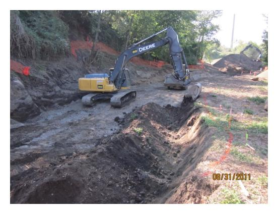
Photo 11. Additional sidewall excavation in Area 1 (delineated by orange paint).
