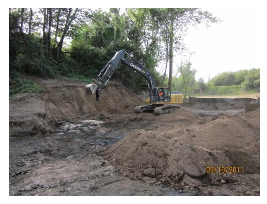
Photo 21. Additional removal of sidewall in Area 2.
