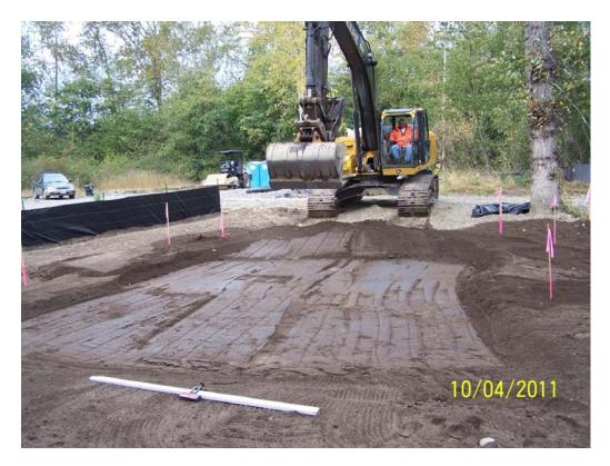
Photo 22. Grading and compacting low-permeable soil for wetland creation.
