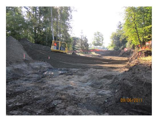
Photo 13. Filling excavation Area 1 with clean sand and gravel.
