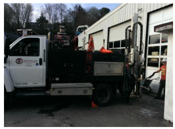
Photograph 1. Installing soil gas point B370.
