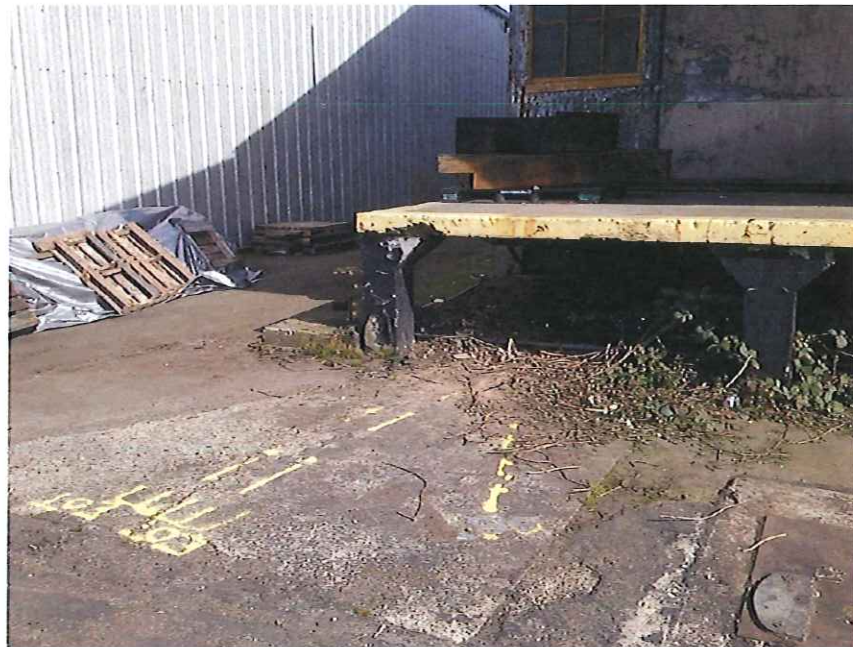
PHOTO 8 - LOOKING NORTHEAST TOWARD LOCATE PAINT OF GROUTED LINES NW OF BUILDING M-19
