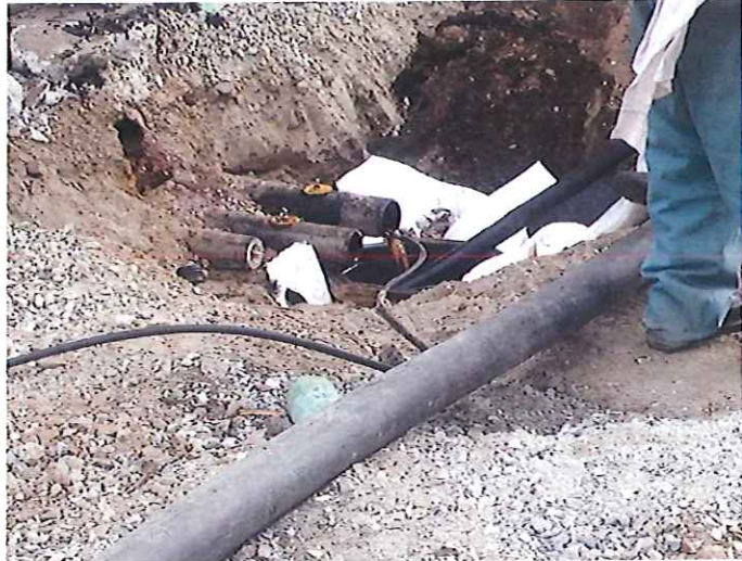
PHOTO 17 - LOOKING NORTHEAST TOWARD THE NORTH TFA BOUNDARY
