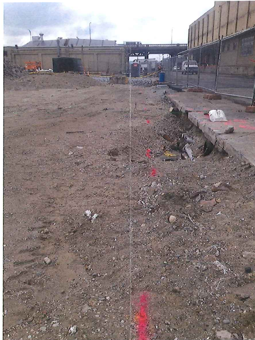
PHOTO 3 - LOOKING SOUTH DOWN COONTZ AVE. TOWARD BUILDING M-28
