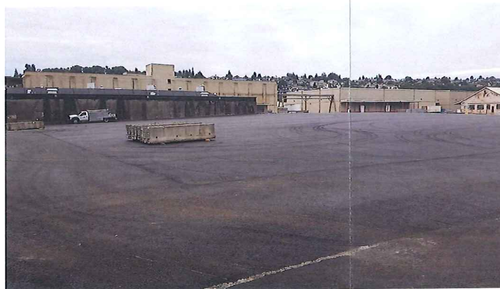
PHOTO 28 - FINAL ASPHALT COVER LOOKING NORTHWEST FROM SE CORNER OF TFA
