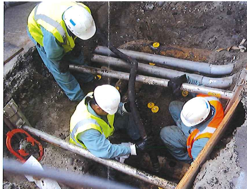
PHOTO 9 - LOOKING SOUTHEAST TOWARD POT HOLE 15
