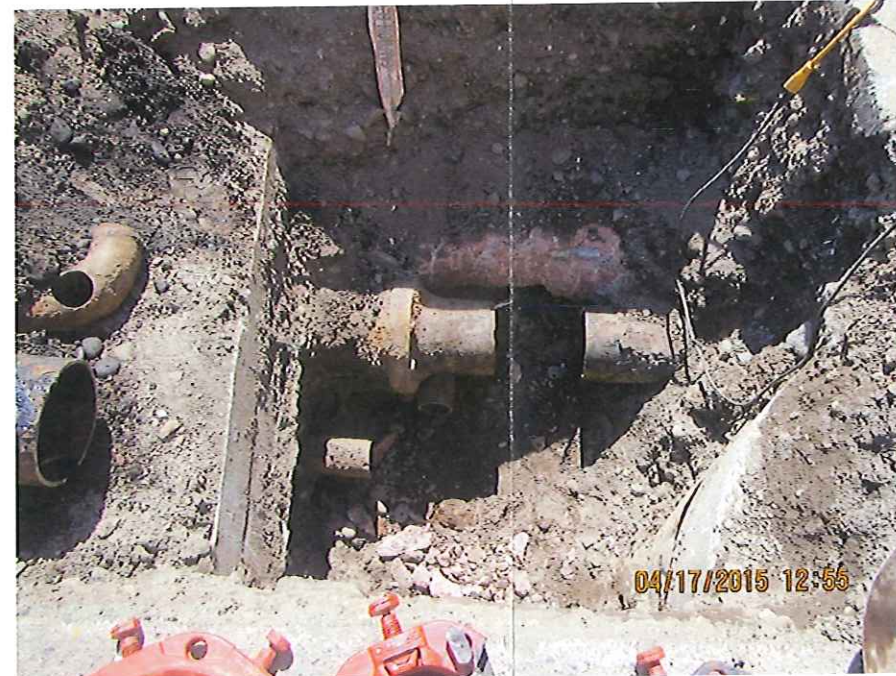
PHOTO 21 - CLOSE UP OF ALLEY POTHOLES PIPES AFTER CUTTING
