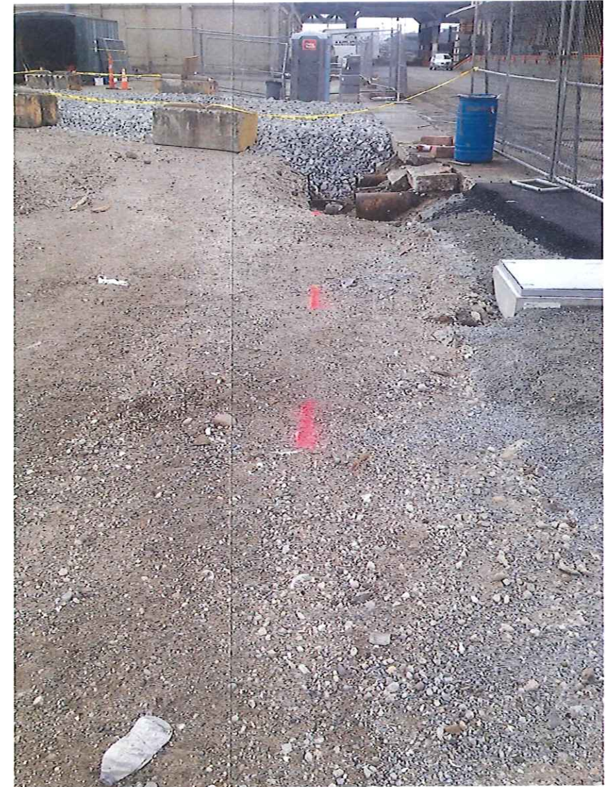
PHOTO 4 - LOOKING SOUTH DOWN COONTZ AVE. TOWARD BUILDING M-28
