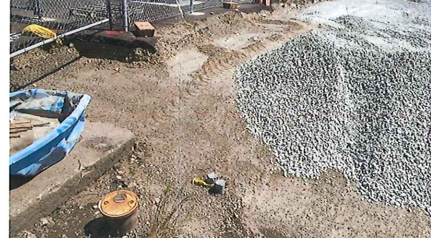
PHOTO 7 - LOOKING NE TOWARDS MWCP_104B AND COMMUNICATION CONDUIT
