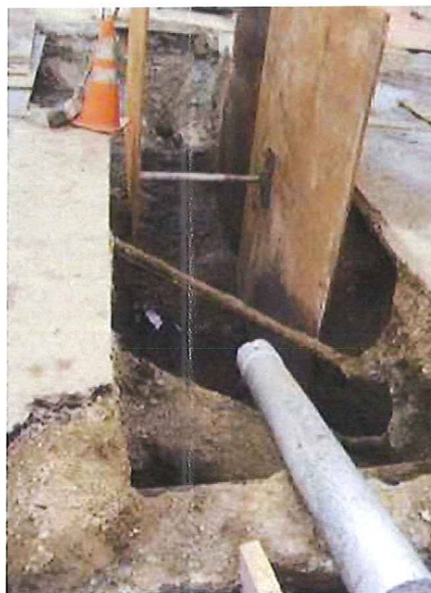
PHOTO 15 - LOOKING EAST AT LNAPL RECOVERY TRENCH 5 DUCT BANK CROSSING
