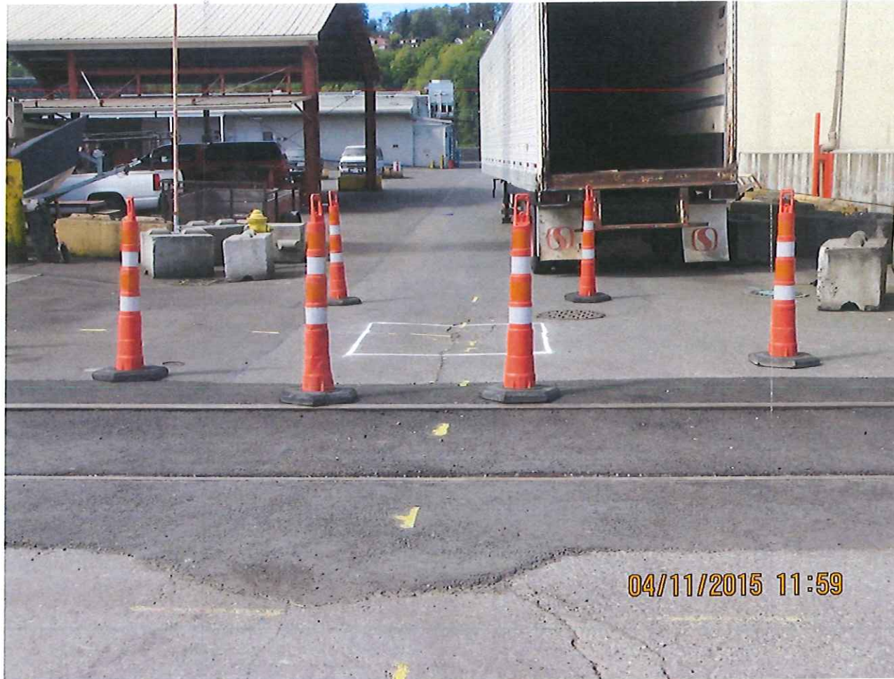
PHOTO 23 - LOOKING WEST TOWARD THE ALLEY POTHOLE LAYOUT PAINT
