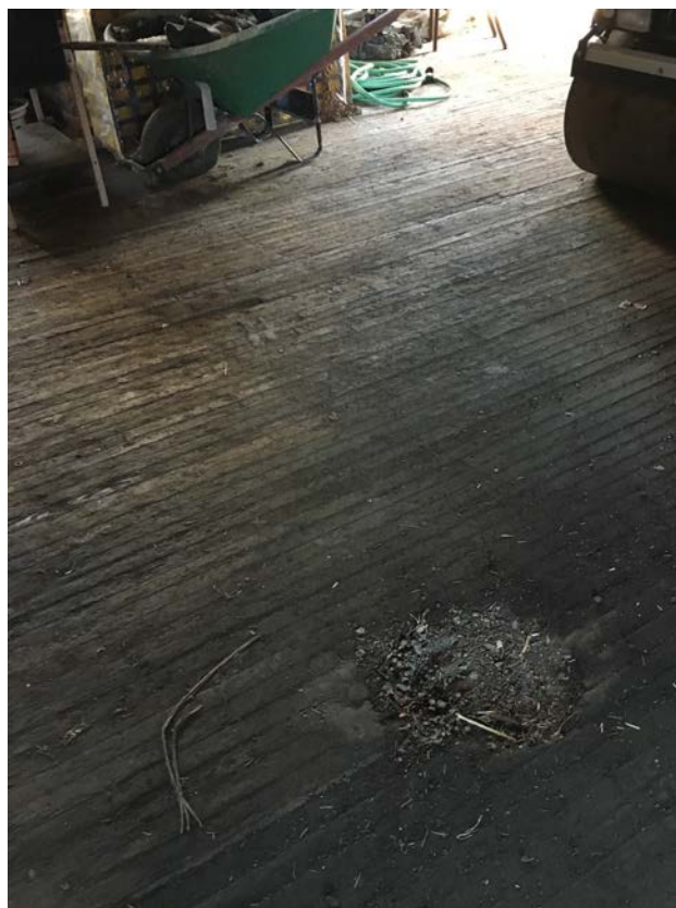
Photo 6: Part of the old shop building has a deteriorated wood floor covering the gravel.
