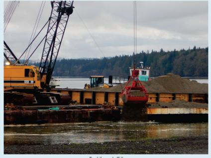
Post-dredging RMC Placement with 9260 Crane and Clamshell Bucket
