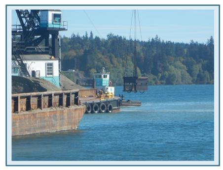
Subtidal Cap Placement in SMA-2 with DB Rainier and Bombay Box
