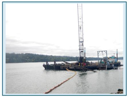
Diver-assisted Removal of Submerged Pilings at the Eastern Wharf
