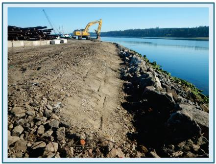
Eastern Wharf – During Asphalt Removal and Armoring
