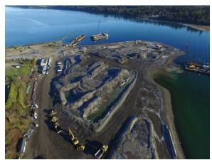
Figure ES-2 – Aerial view of Upland Stockpiles, SMA-1 cap material conveyor, and water-based capping equipment in SMA-1 and SMA-2
