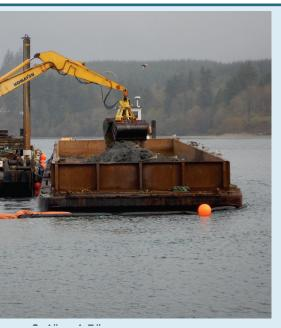
Figure 6 Subtidal Dredging, RMC Placement, and Backfill Buttressing Photographs
