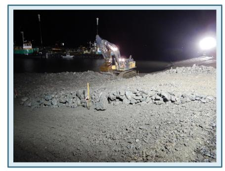
Placement of Type 2 Armor in SMA-1 Intertidal Cap Repair Area
