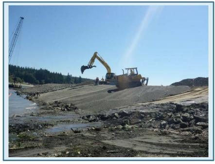
SMA-1 Intertidal Cap Filter Layer Placement
