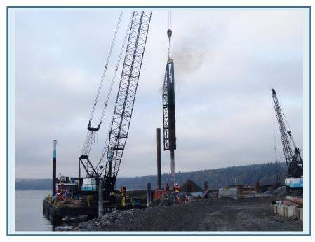
Installation of Temporary Pilings for Transload Extension
