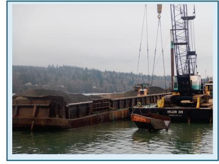
Placement of Angular Gravel Backfill Buttress Material in SMA-2 with 9299 Crane and Skip Box
