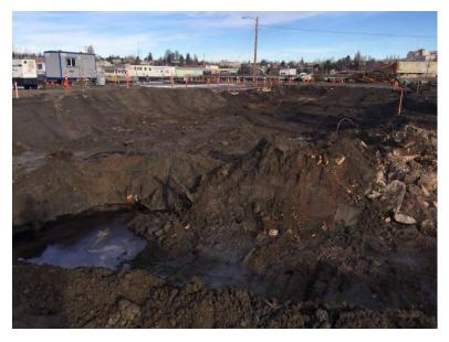
Photograph 4. Overburden removed, contaminated material encountered.
