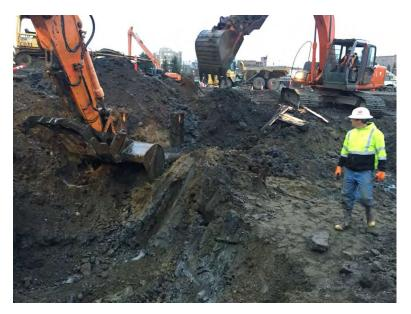
Photograph 7. Excavating contaminated material.
