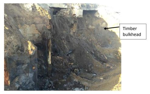
Photograph 9. Excavating contaminated material at bulkhead in NE corner of excavation.
