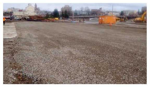
Photograph 12. Finished excavation with top dressing of imported permeable ballast.
