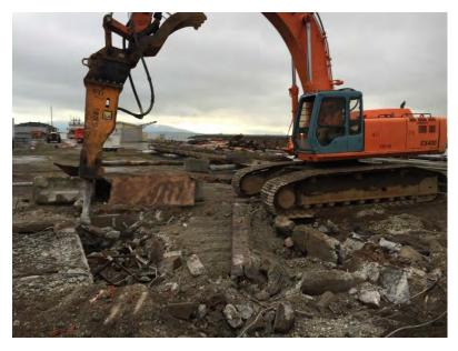
Photograph 1. Removal of surface slab and foundation elements.
