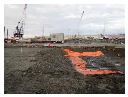
Photograph 11. High-visibility separation geotextile in process of being placed under 2-foot cap of clean import material.
