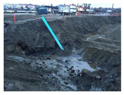
Photograph 5. Dewatering sump in operation.
