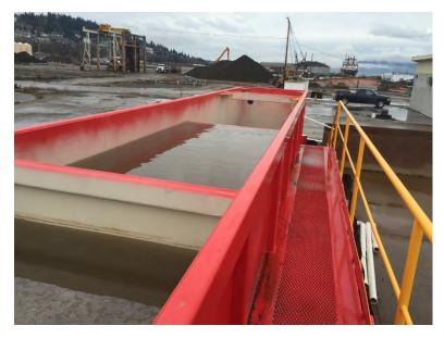
Photograph 6. Weir tank as part of water treatment system.
