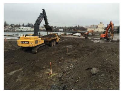
Photograph 3. Loading out of overburden to stockpile area.
