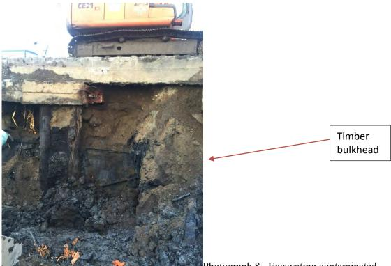
Photograph 8. Excavating contaminated material at bulkhead in NE corner of excavation.
