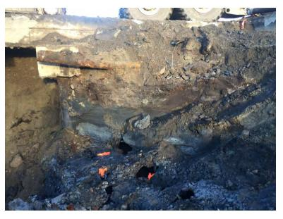
Photograph 10. Excavating contaminated material at bulkhead in NE corner of excavation. Orange flags mark locations of pipes that pierced bulkhead. No evidence of petroleum in pipes. Pipes were cut and capped.
